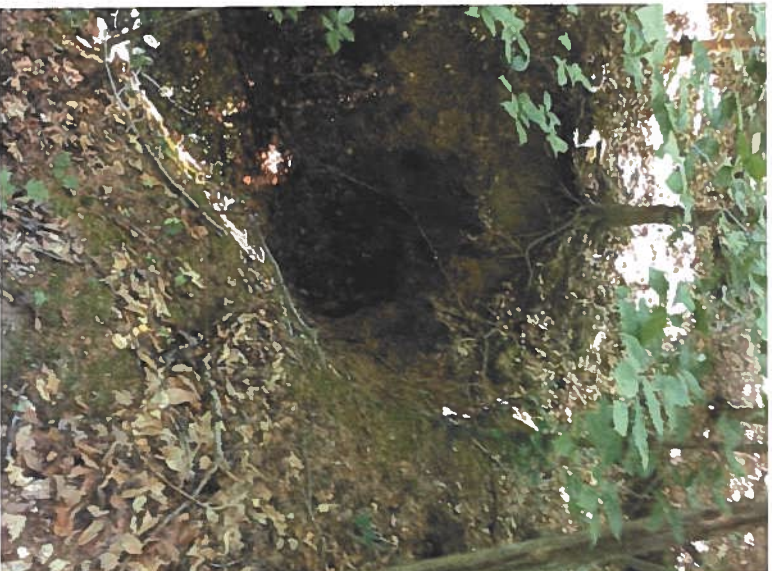
Photograph 2: View of seep and channel.
