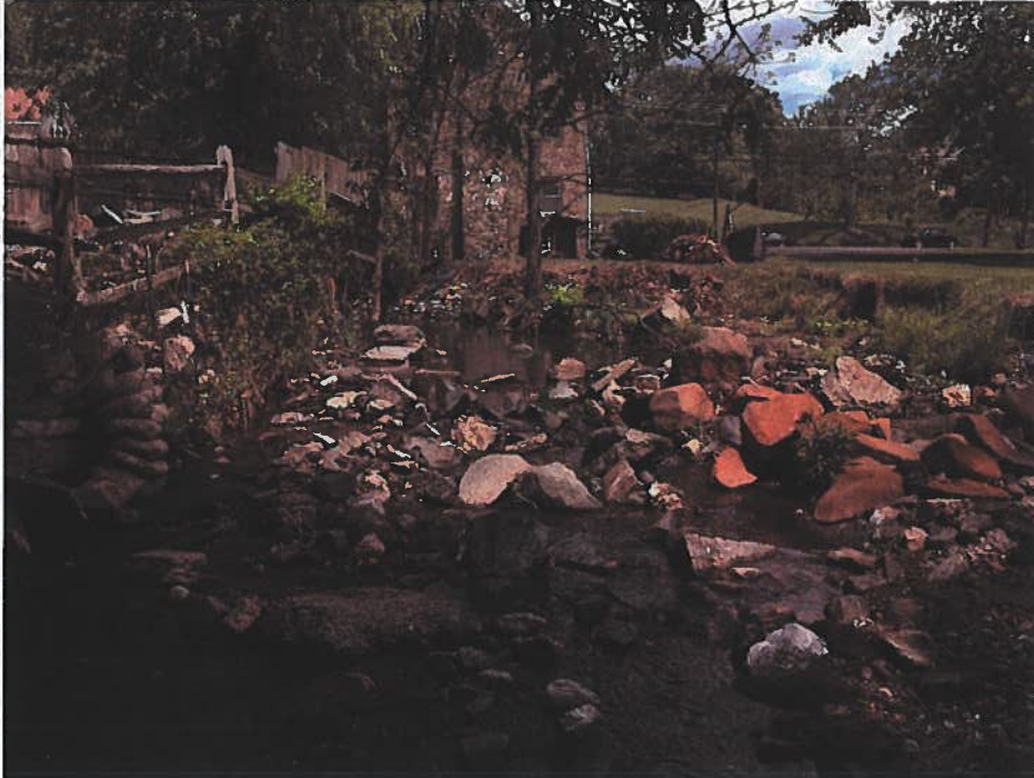
4. Looking upstream at Hudson Branch from the western portion of the study area.
