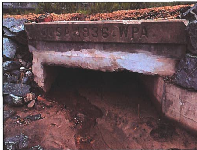
Photo 4: WC3, facing upstream at culvert and confluence of WC3 with WC2
