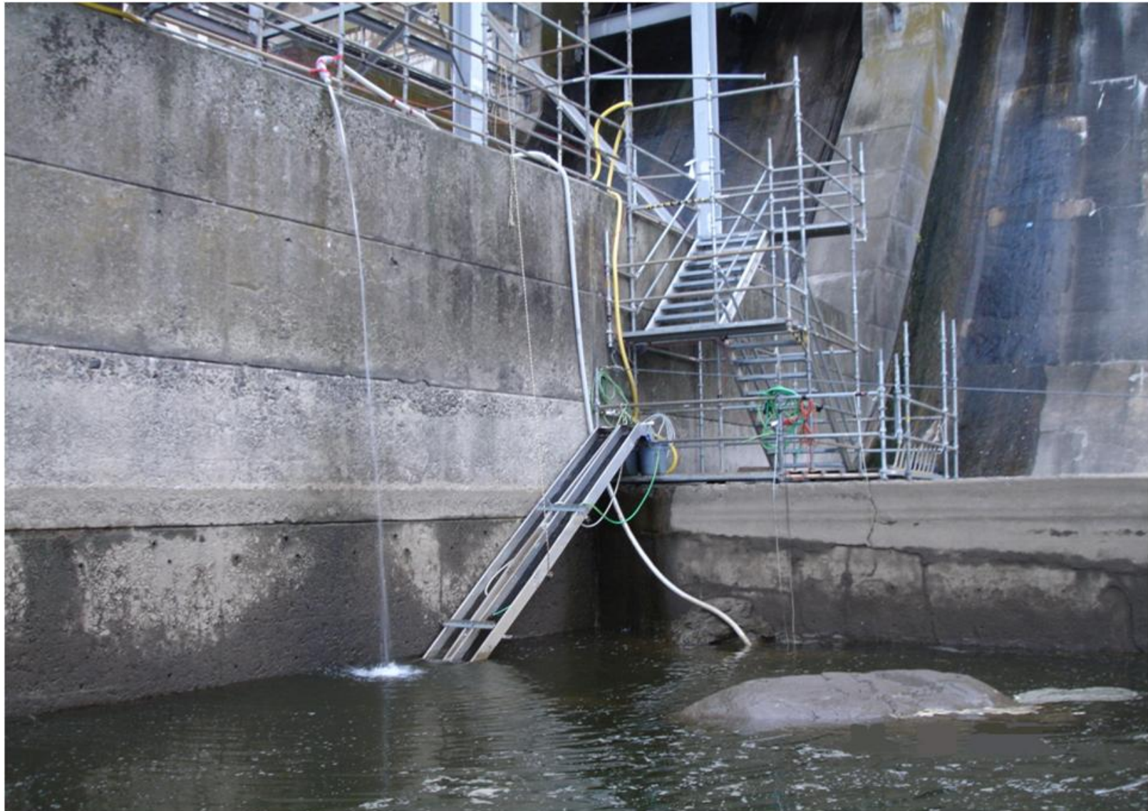
FIGURE 2-3: WEST SIDE ELVER RAMPS WITH ADDITIONAL ATTRACTION WATER.
