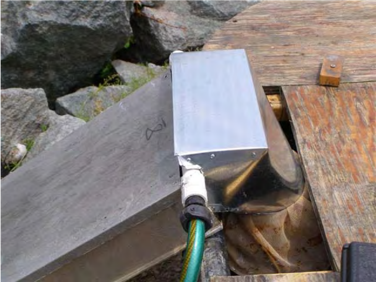
Figure 4. The cable tray emptying into a collection bag in a holding tank.
