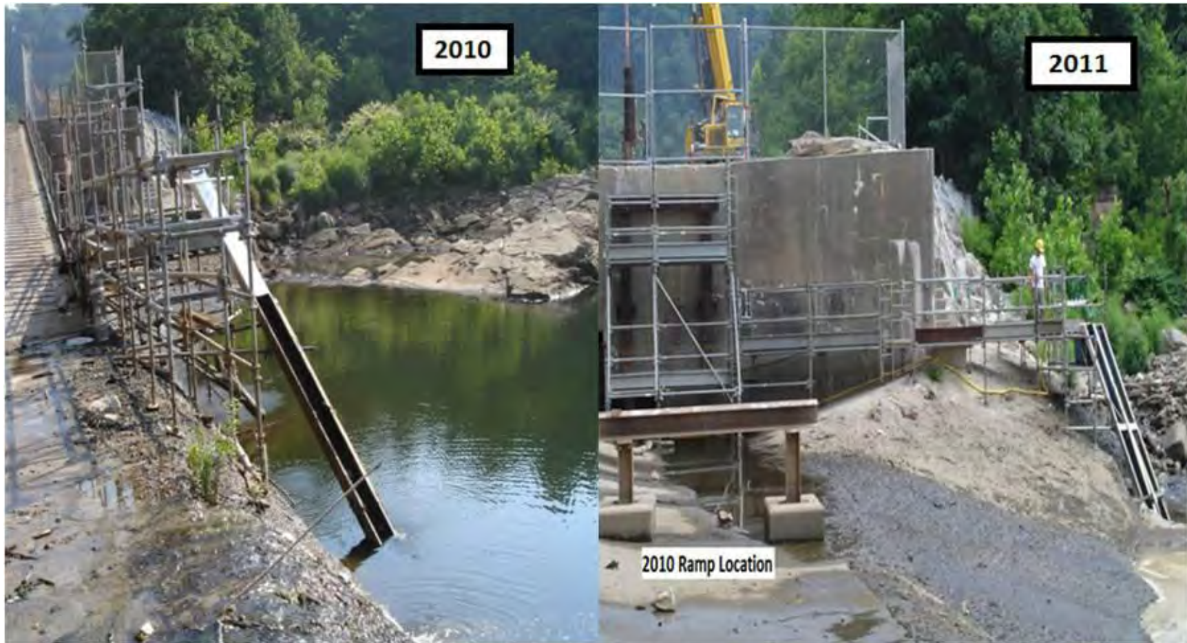
FIGURE 4.3-4: LOCATION AND CONFIGURATION OF EAST SIDE ELVER RAMPS IN 2010 AND 2011.
