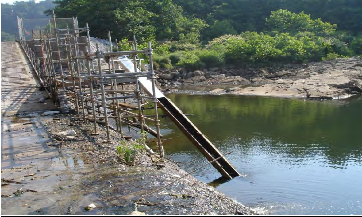
FIGURE 3-4: EAST SIDE ELVER RAMP AT MINIMUM FLOW.
