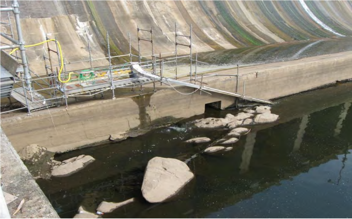
FIGURE 3-2: WEST SIDE ELVER RAMP AT MINIMUM FLOW
