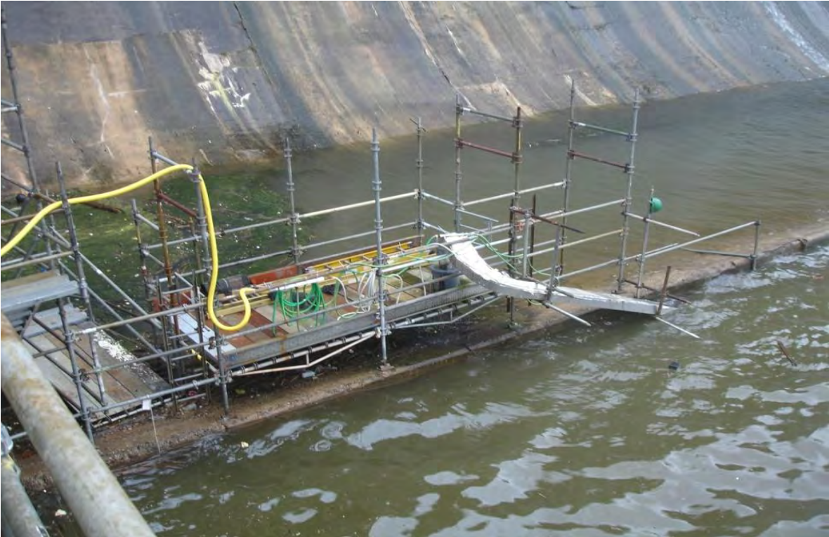
FIGURE 3-3: VIEW OF WEST RAMP DURING FULL GENERATION.
