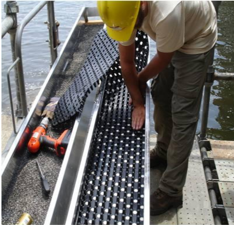
FIGURE 2-7: CONSTRUCTION OF ELVER RAMPS USING TWO DIFFERENT SUBSTRATES.
