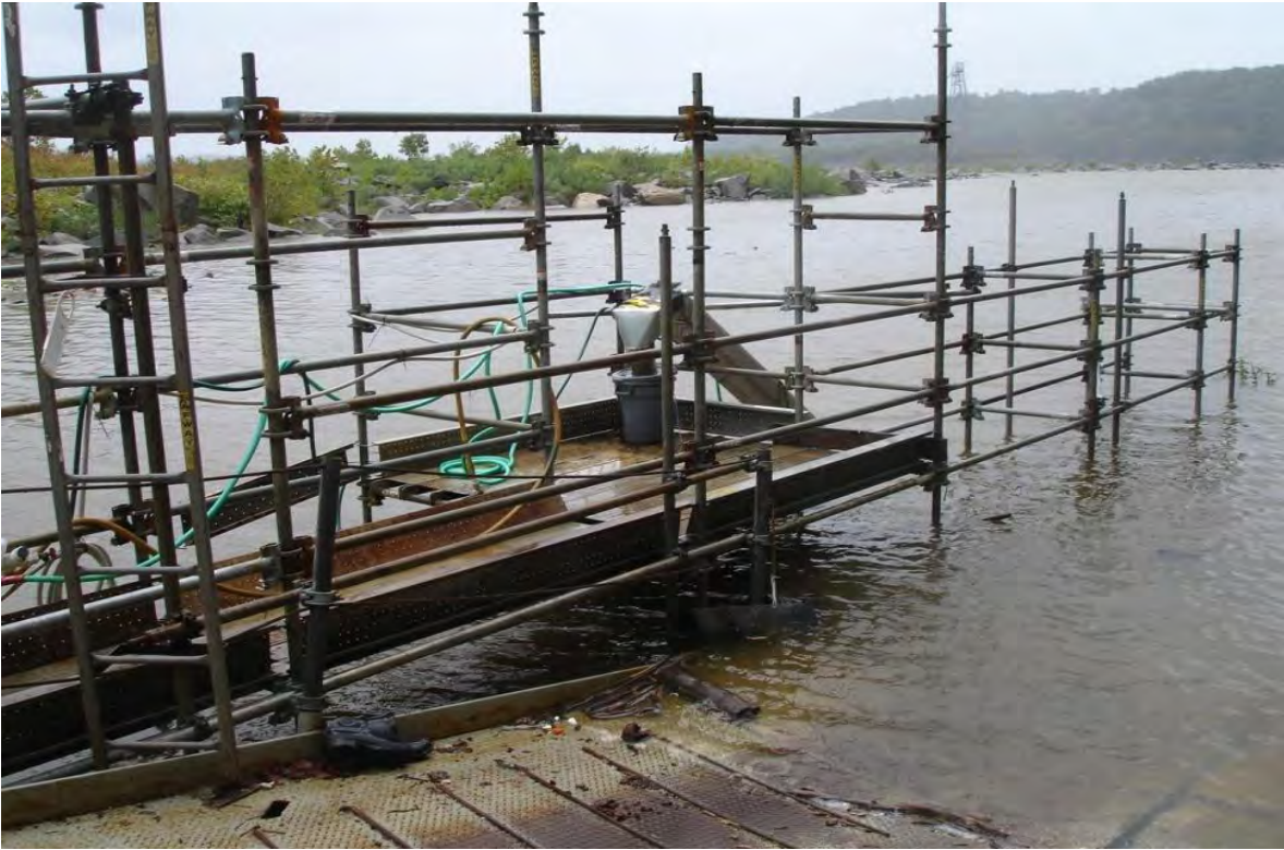
FIGURE 3-5: EAST SIDE ELVER RAMP DURING FULL GENERATION.
