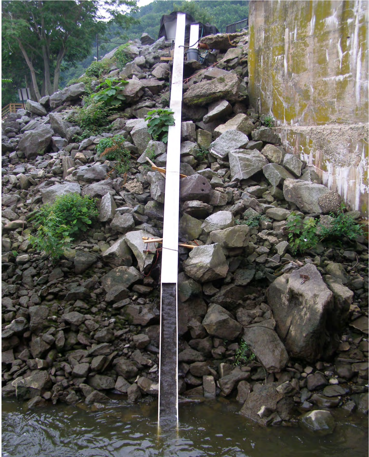
Figure 3. Cable tray on the West Shore below Conowingo Dam, tray on the left is the experimental, and the tray on the right is the control location from 2008.
