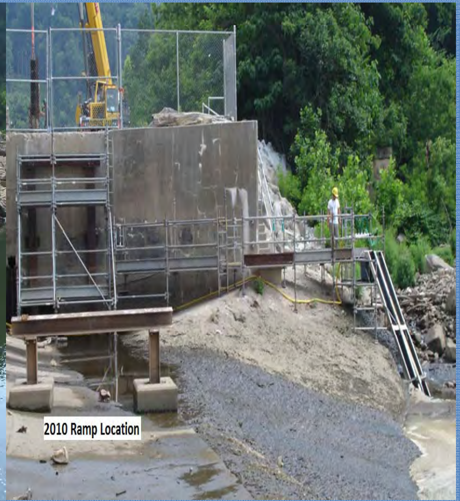
2011 East Ramp Location
