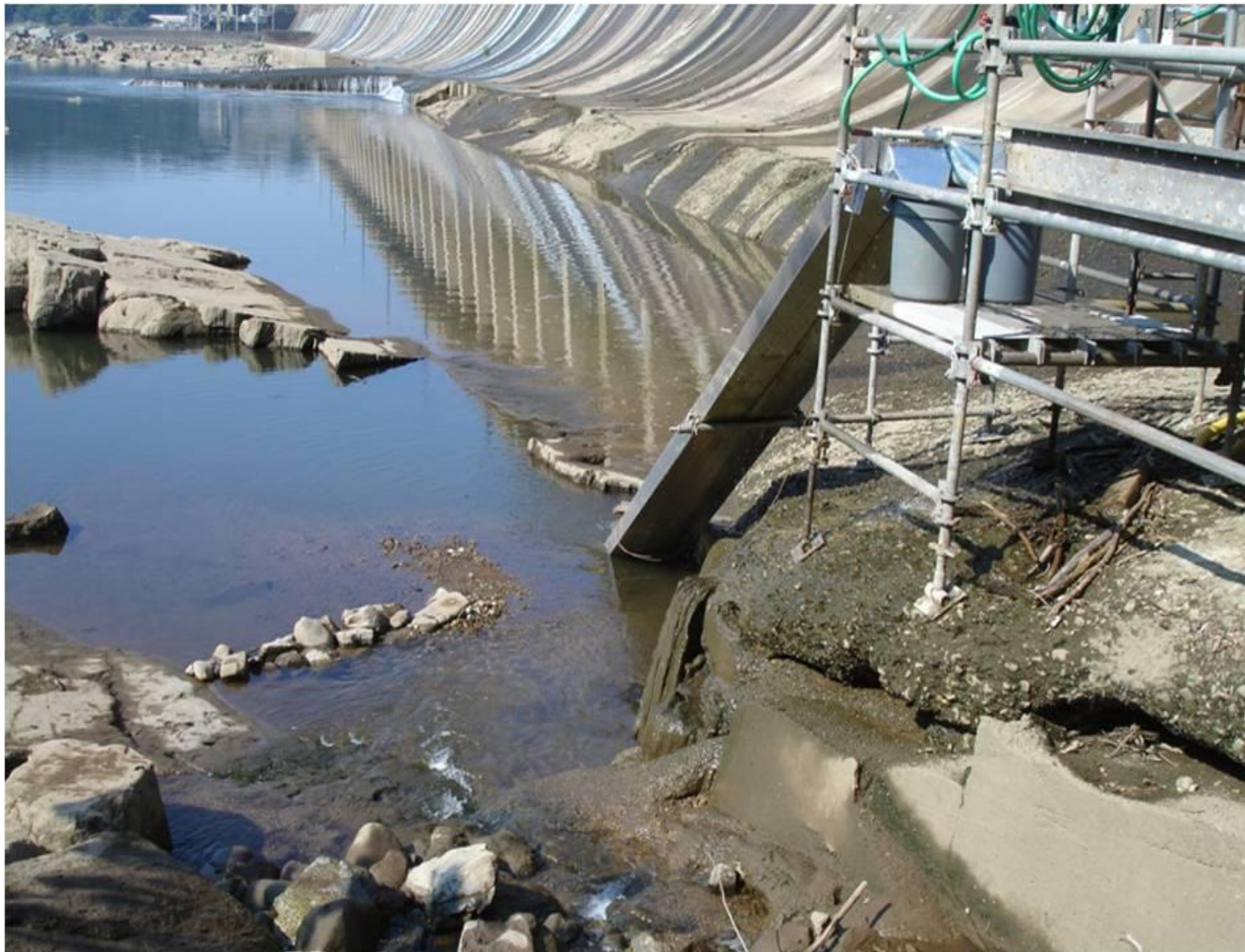
FIGURE 2-6: EAST RAMP WITH NATURAL ATTRACTION FLOW FROM INTERMITTENT STREAM.
