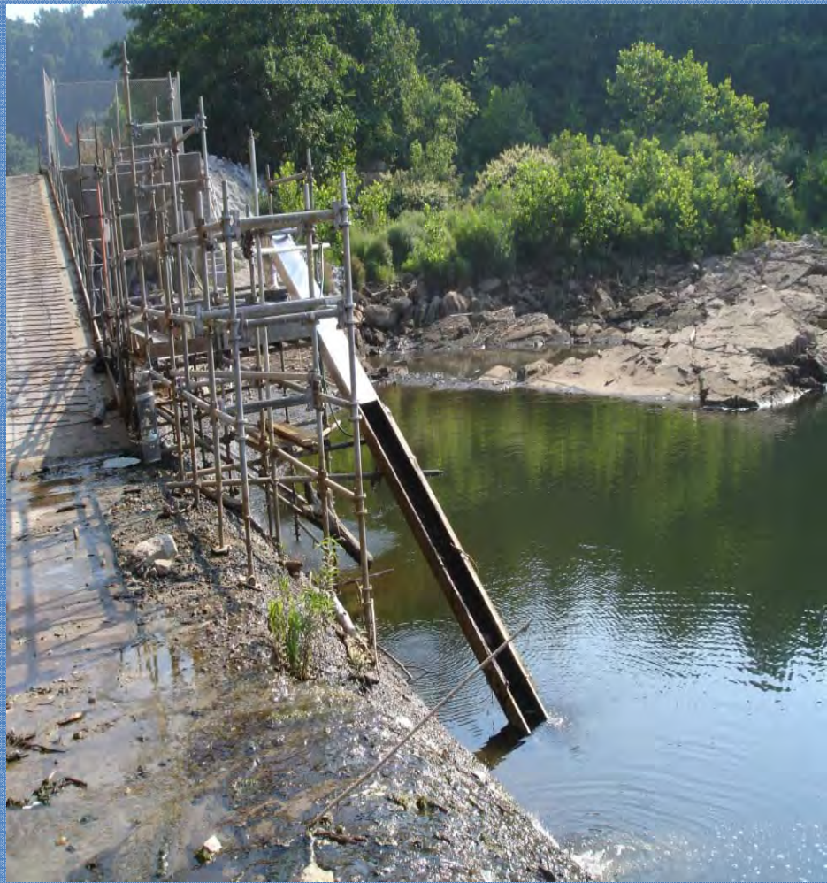
2010 East Ramp Location
