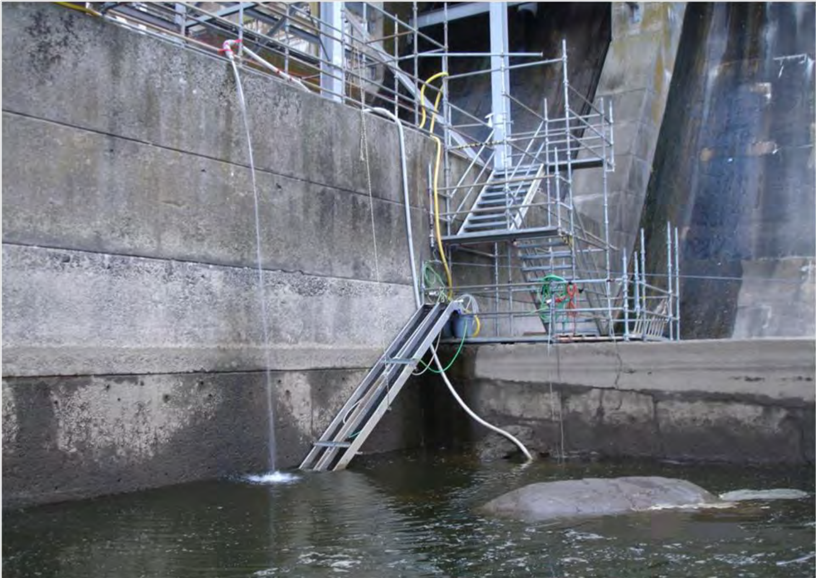
FIGURE 4.3-2: WEST SIDE ELVER RAMPS WITH ADDITIONAL ATTRACTION WATER, 2011.
