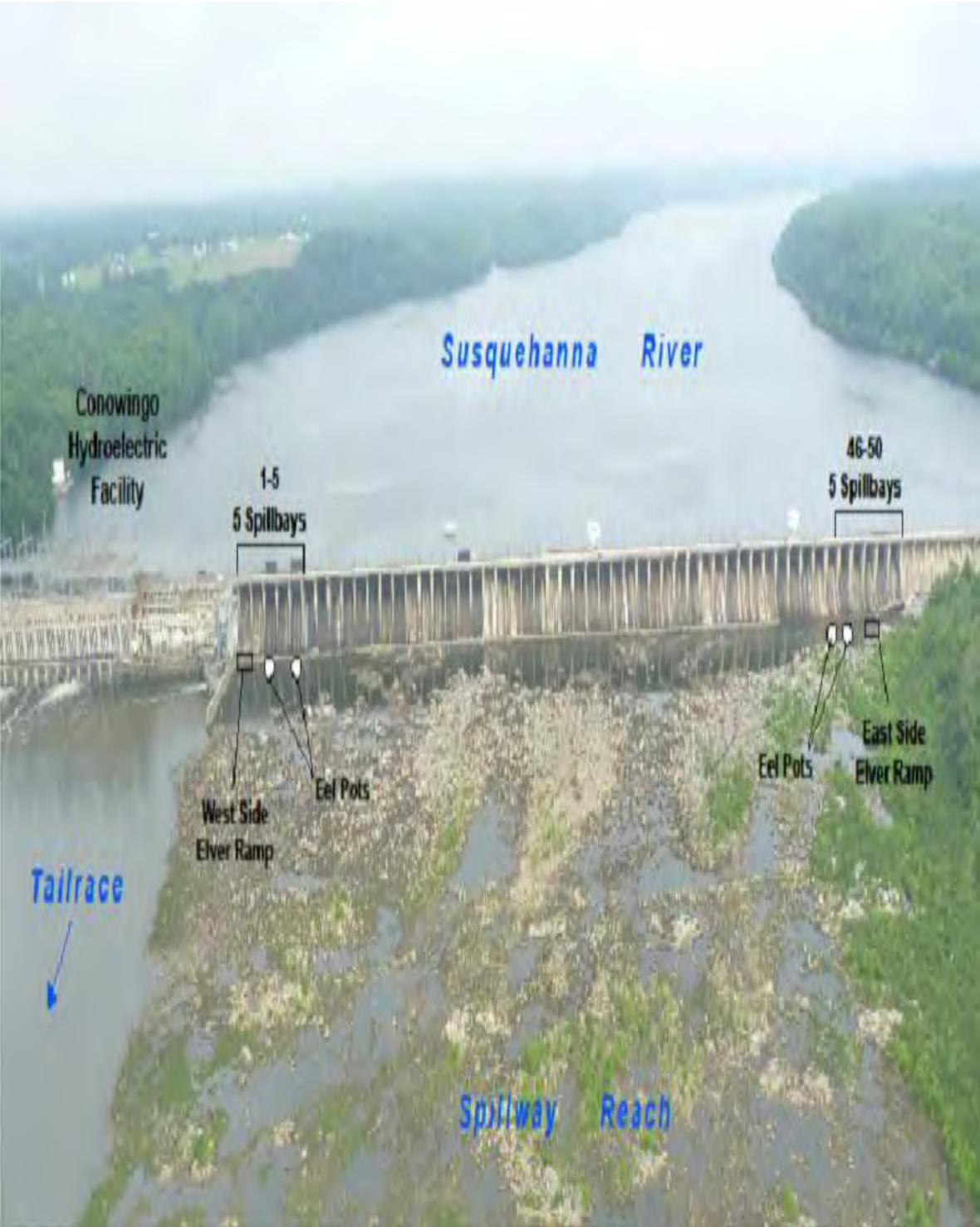
FIGURE 3-1: LOCATION OF ELVER RAMPS AND EEL POTS FISHED IN THE SPILLWAY POOL BELOW CONOWINGO DAM.
