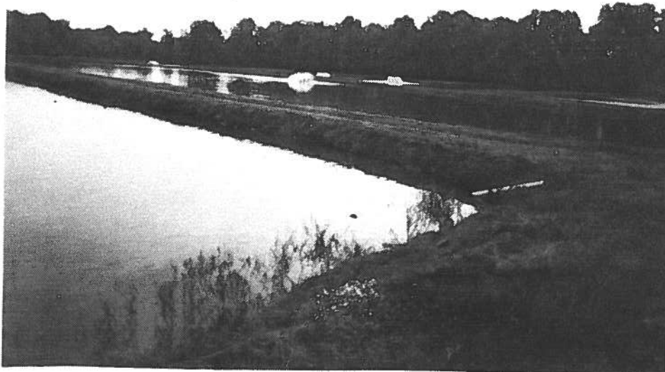
View of some of the many fish hatchery ponds found in the Fishing Creek watershed. Most of these are privately owned. The woodline in the background of this photo is actually the left bank (looking downstream) of Fishing Creek. Though some (relatively few) of these embankments are expected to be overtopped by the 100 year flood, resulting in a loss of the enclosed fish, the structures themselves should see only minor damage due to the shallow depths and low velocities anticipated in this vicinity. Since these are dugout ponds there is no hazard potential should failure occur.
