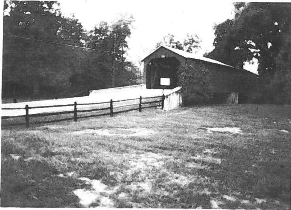
The covered bridge on Utica Road is of historical value. Though the approaches to this bridge will be inundated by the 25 year flood the structure itself is perched above the 100 year flood.
