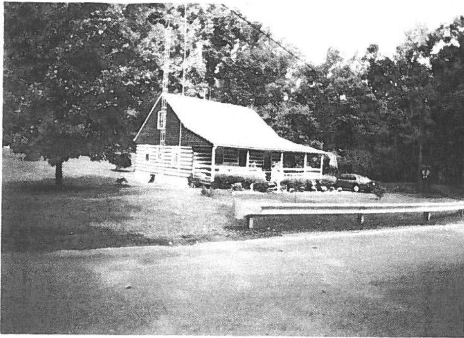
Typical of the many cabins found in the upper Fishing Creek Watershed. Some of these are expected to sustain damage during the 100 year flood.
