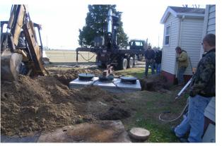
Connection of the waste stream to a wastewater treatment plan
