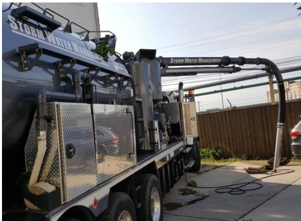
Storm drain vacuuming
