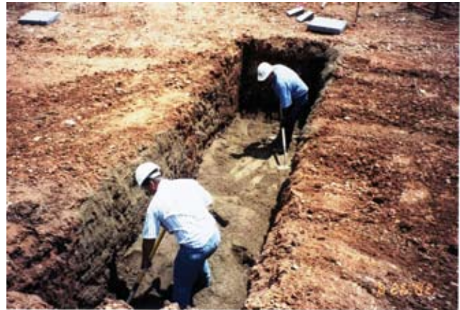
(b) Filter diaphragm trench excavated and backfilled with sand
