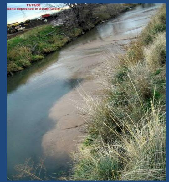
Significant sediment deposition in South Drain
