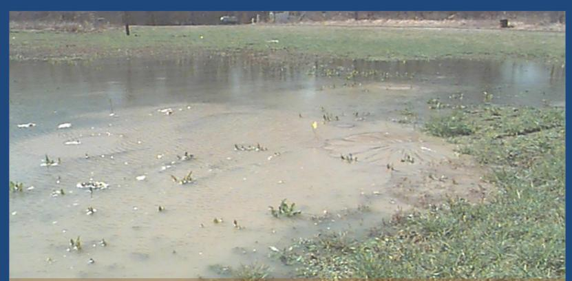
Sand boils just beyond downstream toe of embankment with substantial seepage through the foundation collecting along the downstream area. No drain to intercept seepage.
