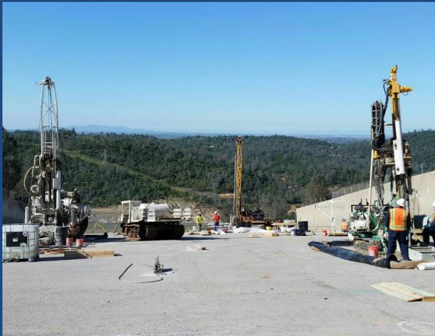
Condition of Remaining Chute
