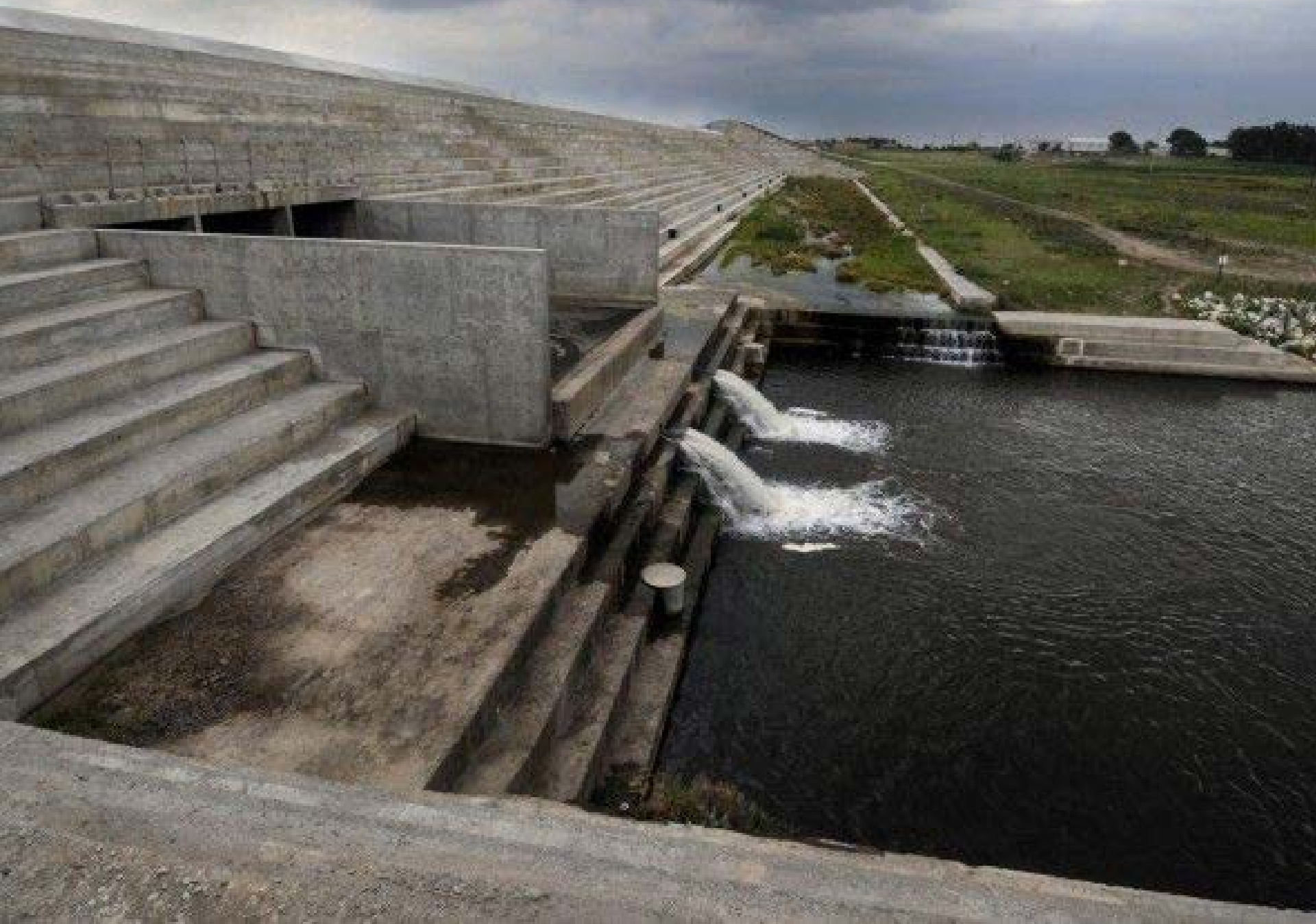
Lake Wanahoo Spillway
