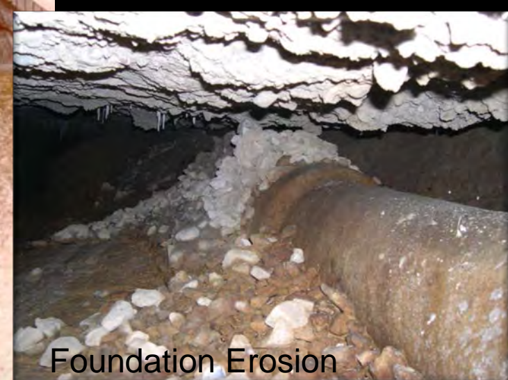
Slab Failed in 1983 After 30 years of Operation
