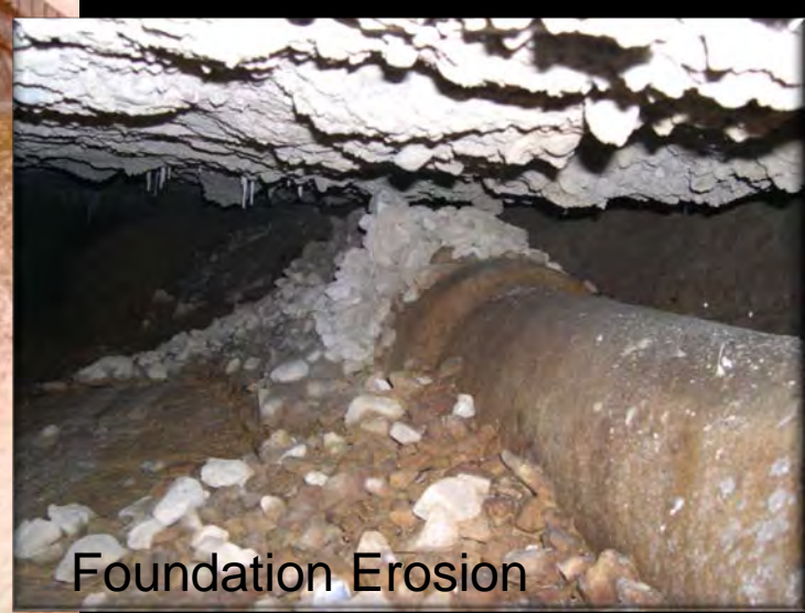
Slab Failed in 1983 After 30 years of Operation
