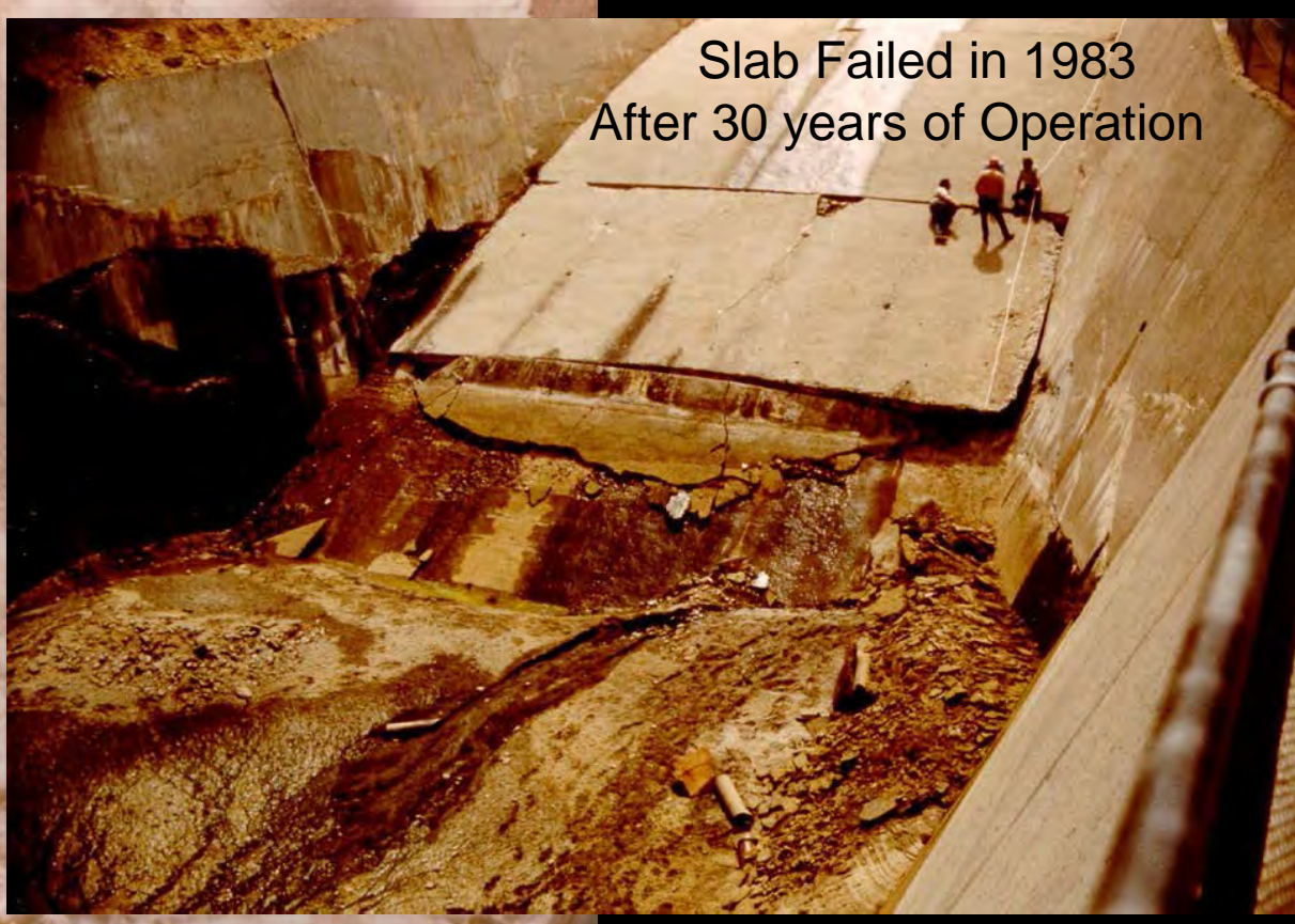
Foundation Erosion
