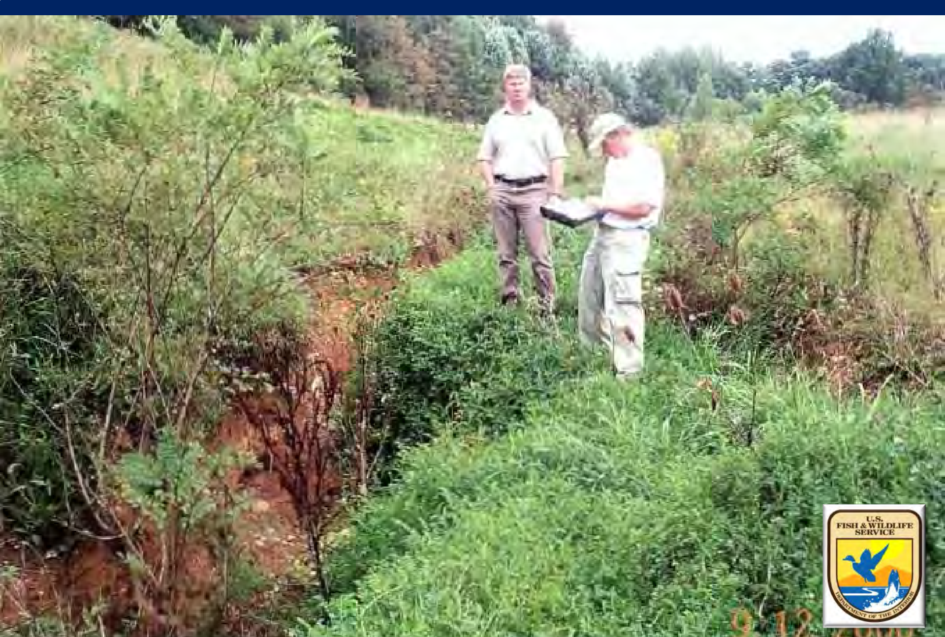
28. Erosion gully in downstream channel of emergency spillway, looking upstream. Old Timbers Dam, Big Oaks NWR, Indiana
