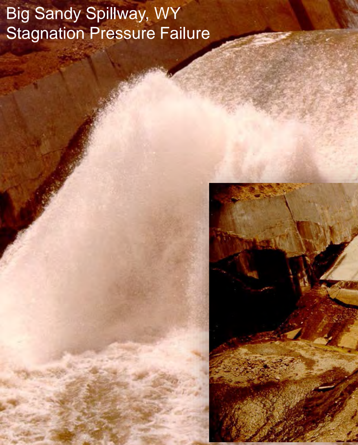
Slab Failed in 1983 After 30 years of Operation
