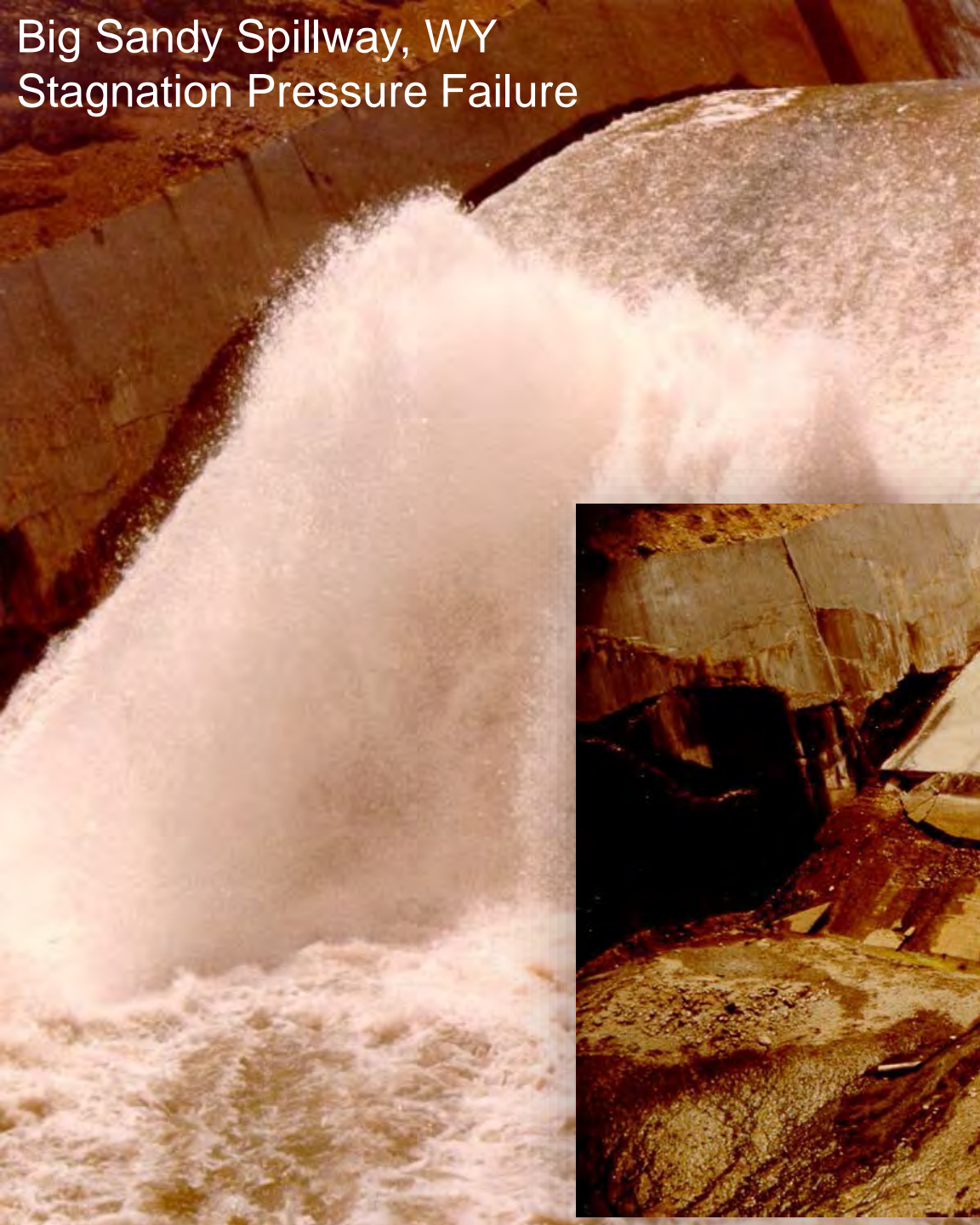
Foundation Erosion
