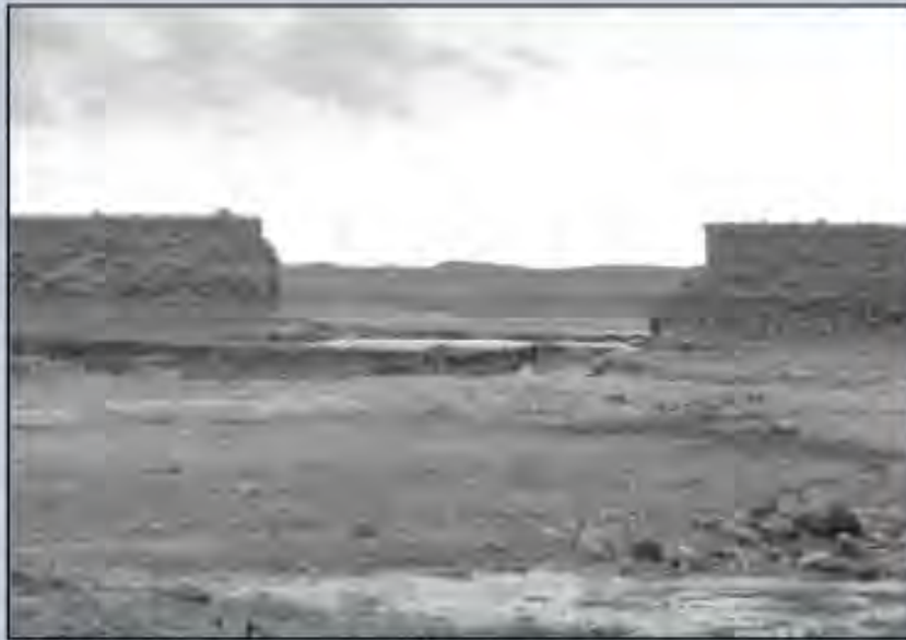
Taylor Creek Dam Failure - Photo by Candace Linder, NRCS
