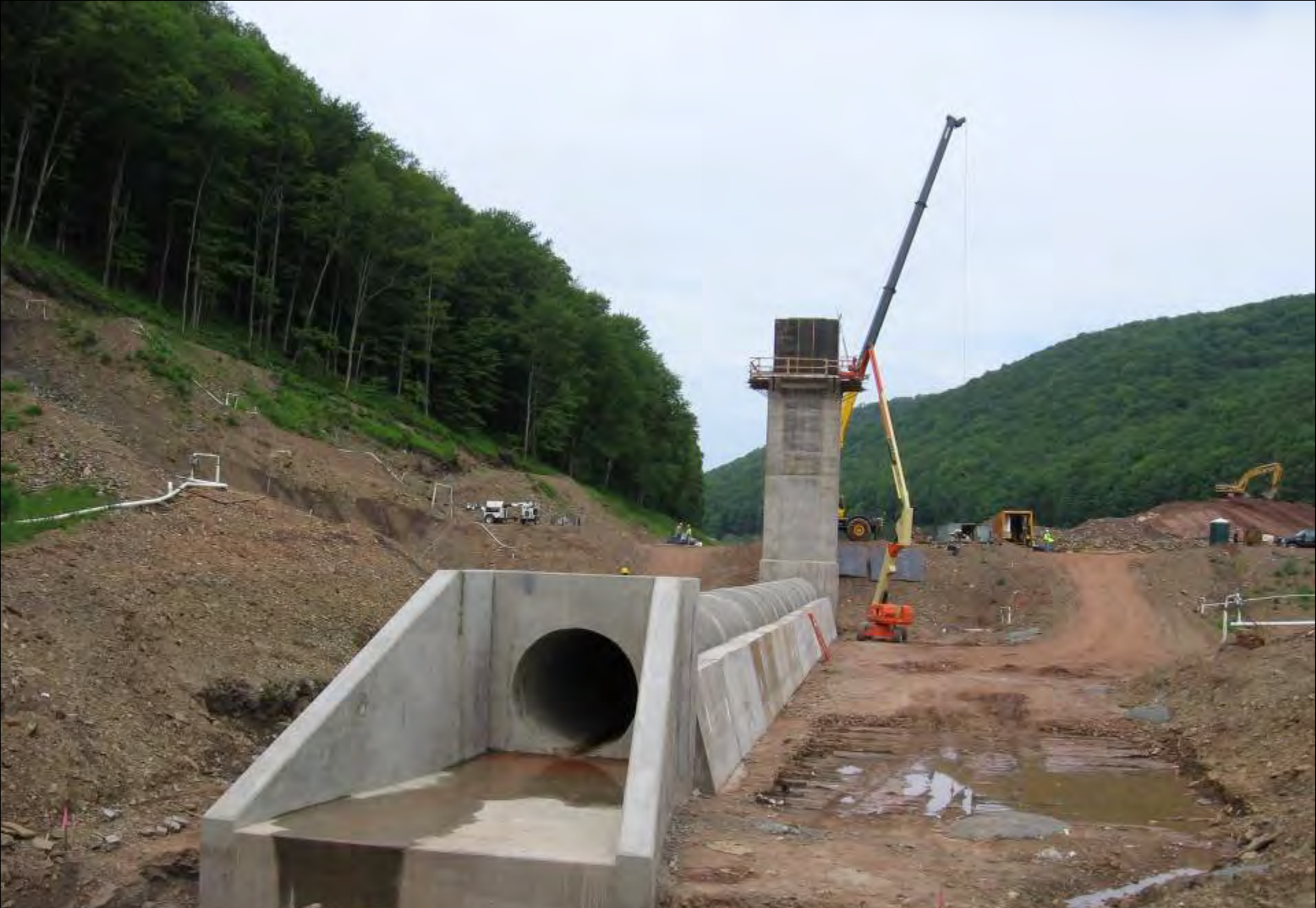
8' Diameter RCP & Outlet Structure. View Looking Upstream
