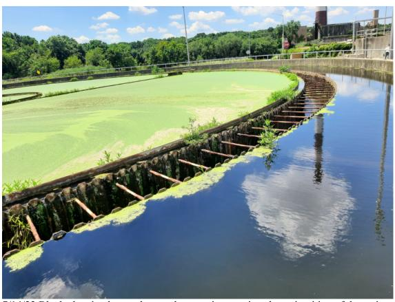
7/14/22 Blocked weirs due to algae and vegetation causing short circuiting of the weirs.
