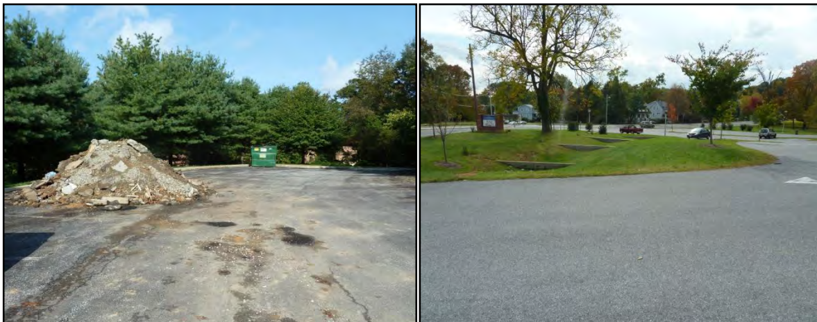
Figure 4-31: Unprotected Stockpile at ISI_C_402 (left) and Existing Dry Grass Swale at ISI_C_403 (right)
