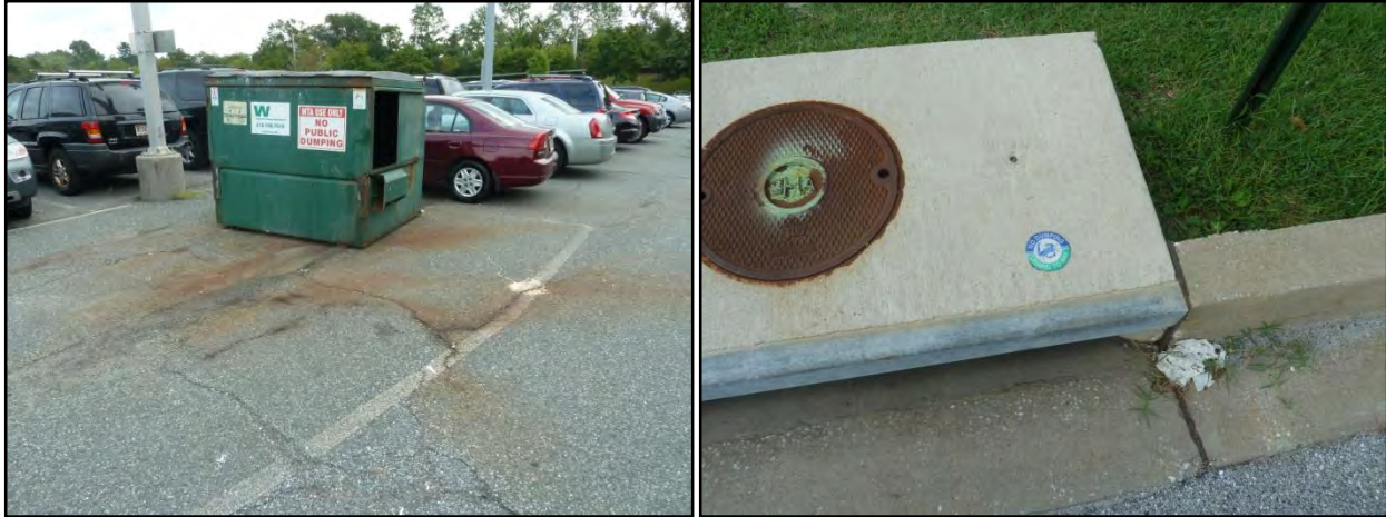
Figure 4-4: Leaking Dumpster (left) and Storm Drain Marking (right) at HSI_C_102
