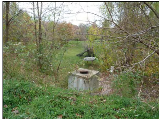
Figure-4-32: Pond Embankment (left) and Control Structure with Missing Lid (right) at Detention Pond SWM_C_859
