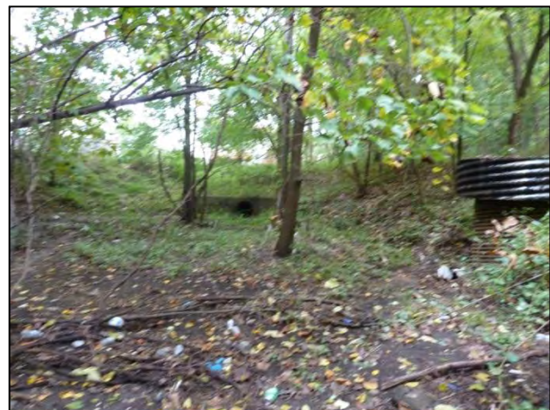
Figure 4-11: Impervious Access Road (left) and Trees, Trash near Riser (right) at SWM_C_441
