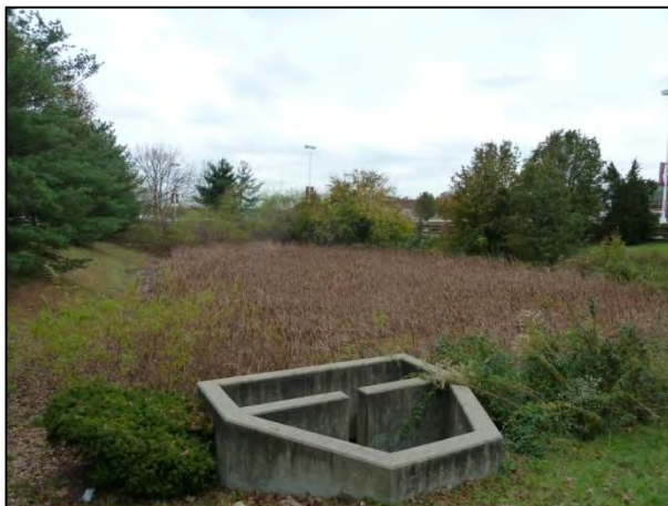
Figure-4-26: Dense Invasive Vegetation Around the Outlet Structure (left) and Curb Cut Inlet Configuration (right) Draining to SWM_C_857
