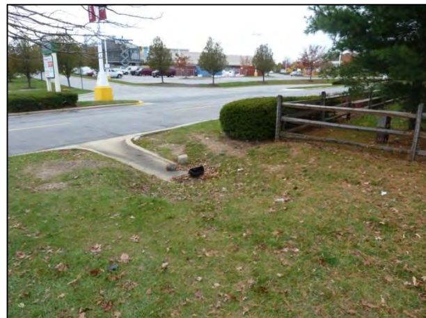
Figure-4-26: Dense Invasive Vegetation Around the Outlet Structure (left) and Curb Cut Inlet Configuration (right) Draining to SWM_C_857
