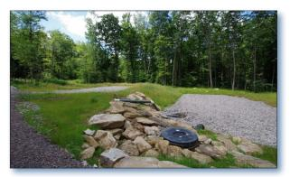
Figure 2. Limestone leach bed, installed in 2014 in the headwaters of Big Laurel Run.
