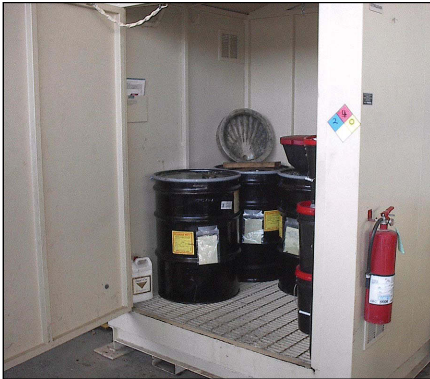
Figure 5. Minimize exposure by providing cover for potential contaminants.
