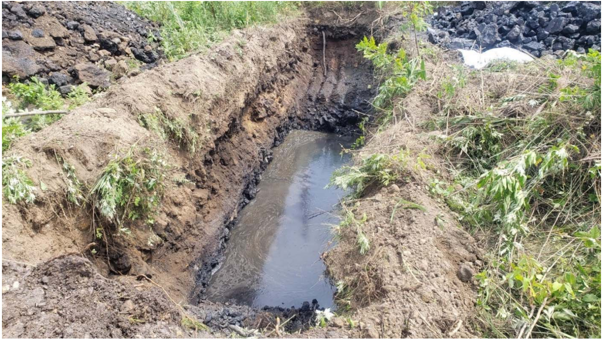
070821-6: TP-4 – Test Pit following excavation
