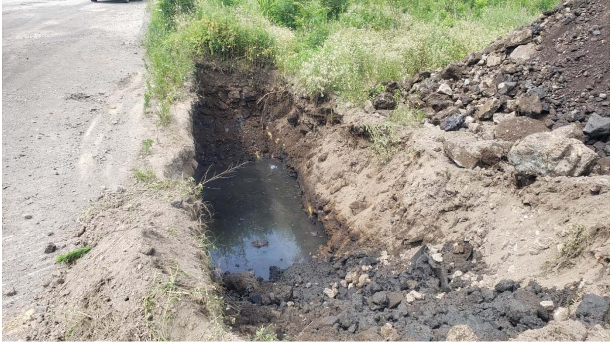
070821-4: TP-3 – Test Pit following excavation
