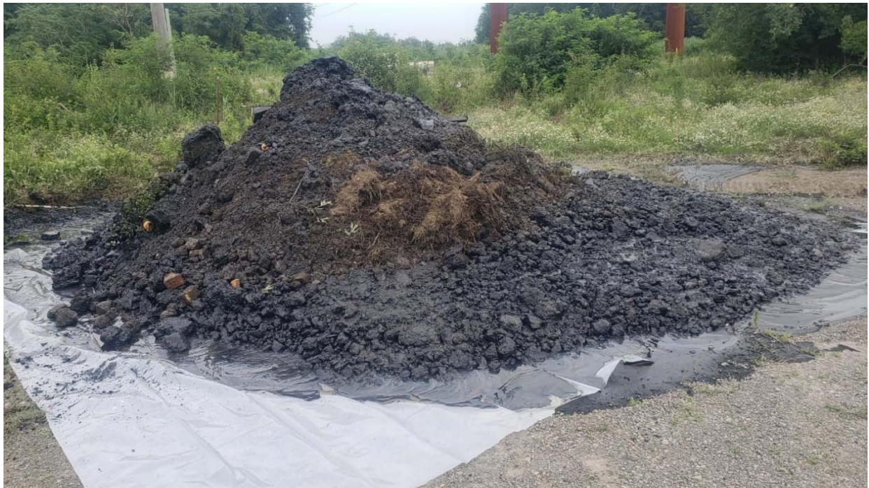
070821-3: TP-2 – Excavated Material Stockpile
