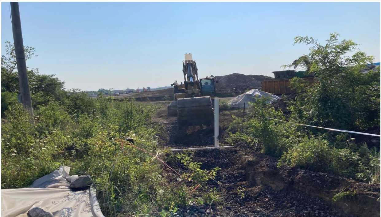
080621-2: TP-2 – Temporary Monitoring Point (Backfilled)
