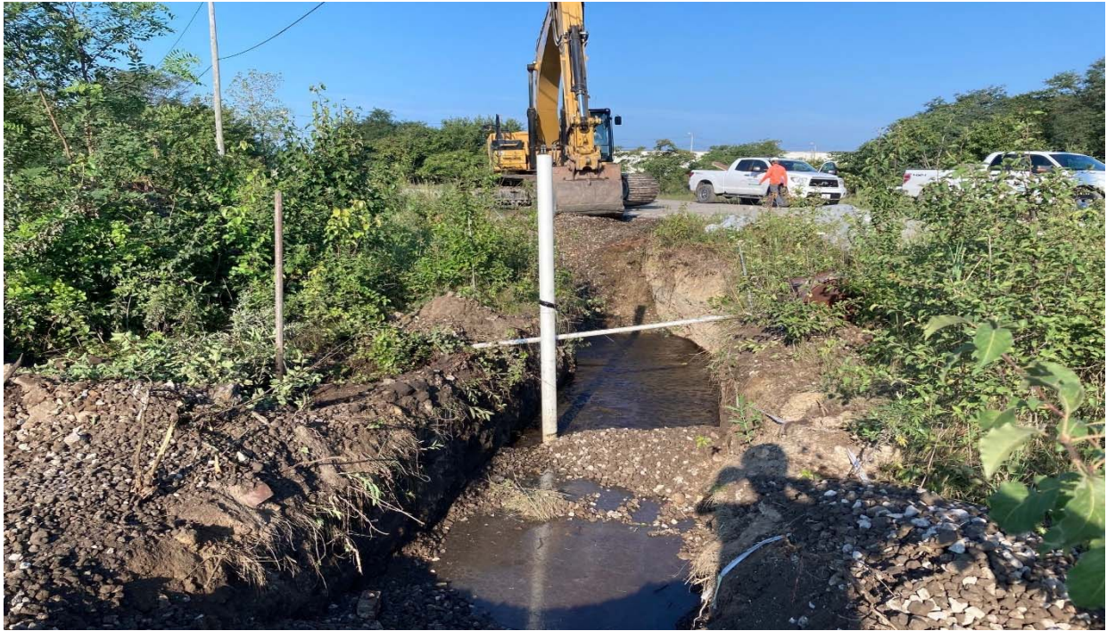
080621-1: TP-2 – Observation Point (While Backfilling)
