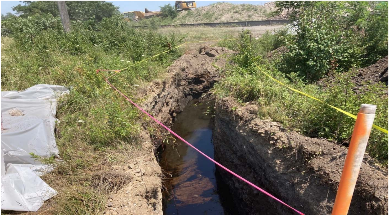
071221-1: TP-2 – Test Pit following extraction
