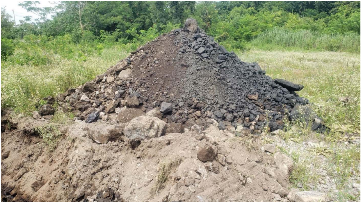
070821-5: TP-3 – Excavated Material Stockpile
