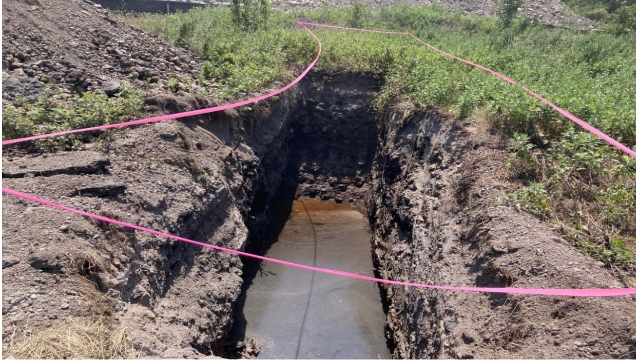
070821-1: TP-1 – Test Pit following excavation
