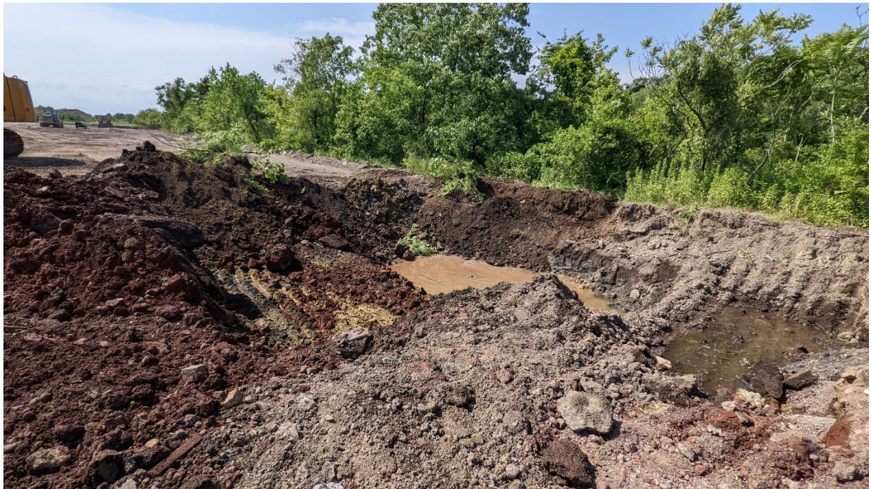
Photo 4: Response Area A11-024CC-SB, facing north
