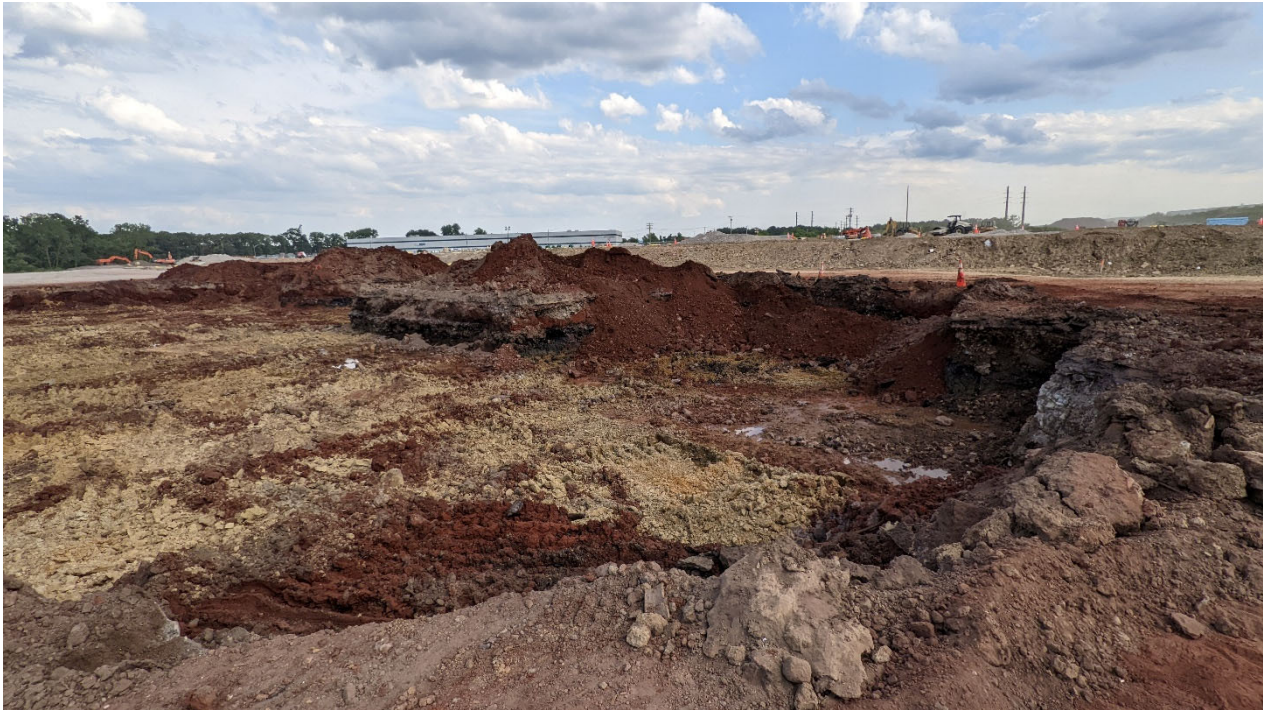
Photo 6: Response Area A11-024H-SB, final excavation area, facing south
