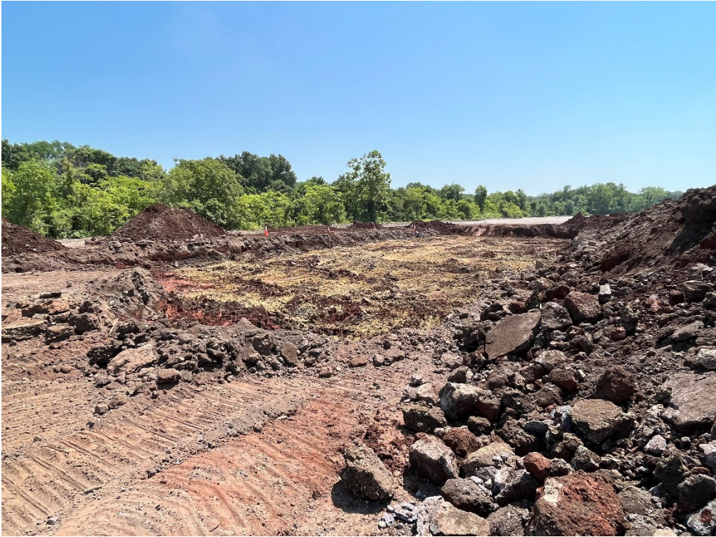
Photo 7: Response Area A11-024H-SB, excavation area, facing east
