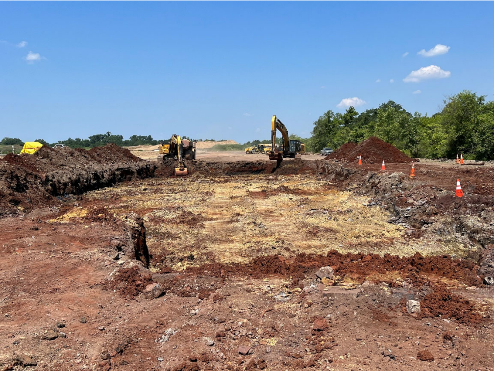
Photo 8: Response Area A11-024H-SB, excavation area, facing northwest
