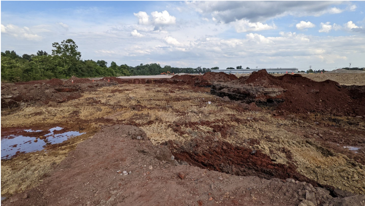
Photo 5: Response Area A11-024H-SB, final excavation area, facing east
