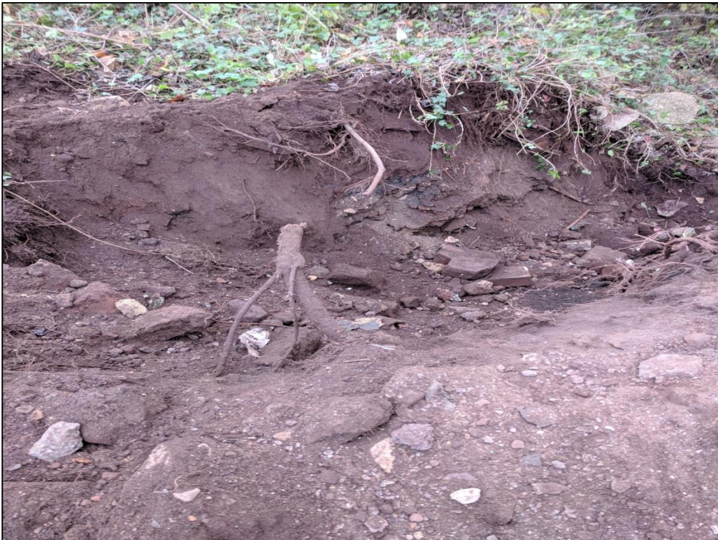
Photo 4: View of the completed A5-002-TP. Fine to coarse grained soils (silt, sand, and gravel) and slag fill materials were observed. PID reading of 3.3 ppm was recorded.
