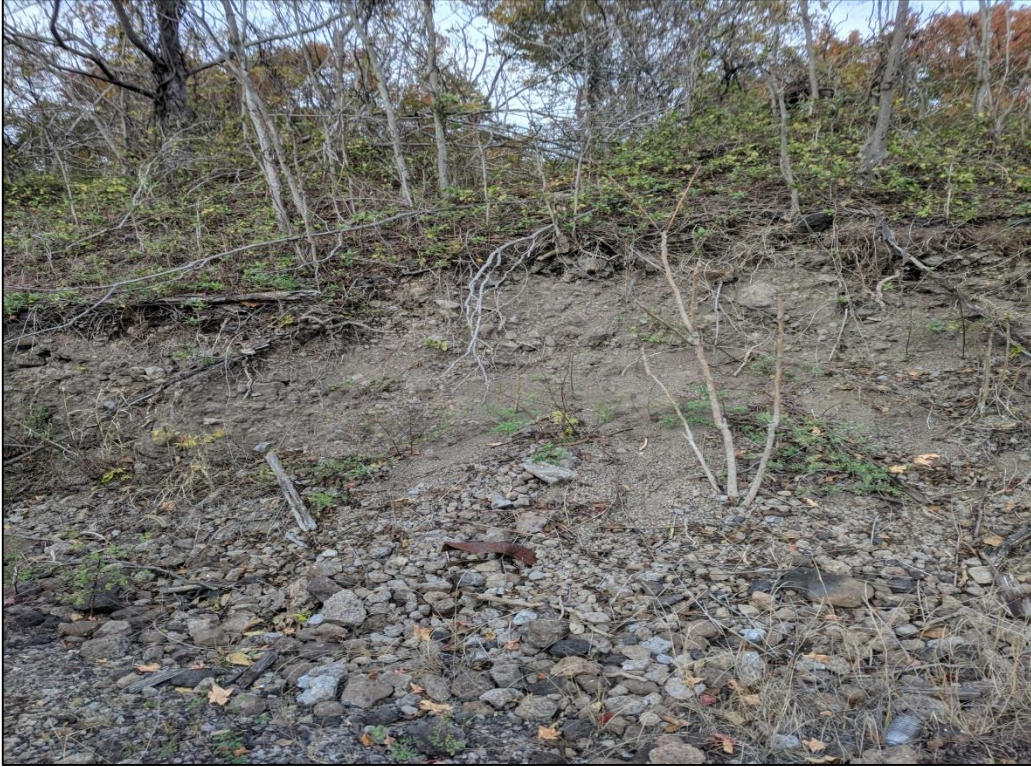
Photo 17: View of GRY-001-TP prior to excavation activities from the bottom of the berm. View is from the south facing north.
