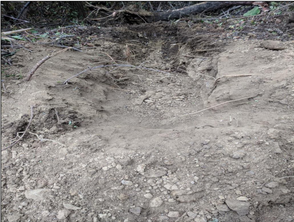
Photo 16: View of A5-008-TP after excavation activities. Fine to coarse grained soils (silt, sand, and gravel) and slag fill materials were observed. A PID reading of 4.2 ppm was recorded.
