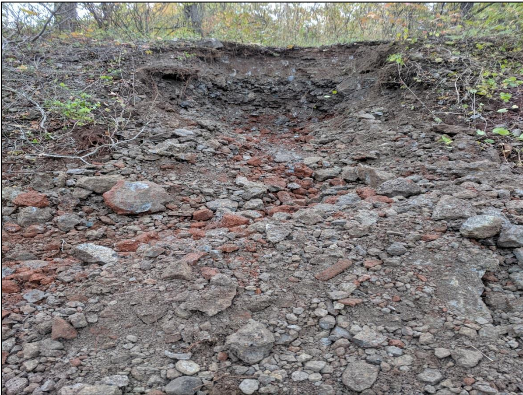
Photo 12: View of A5-006-TP after excavation activities. Fine to coarse grained soils (silt, sand, and gravel) and slag fill materials were observed. A PID reading of 5.1 ppm was recorded.
