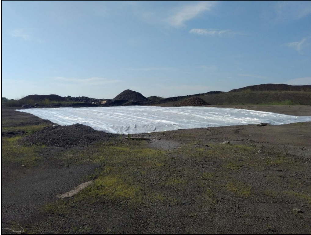
07/16/19-3: View to the southwest of the stockpile holding area.
