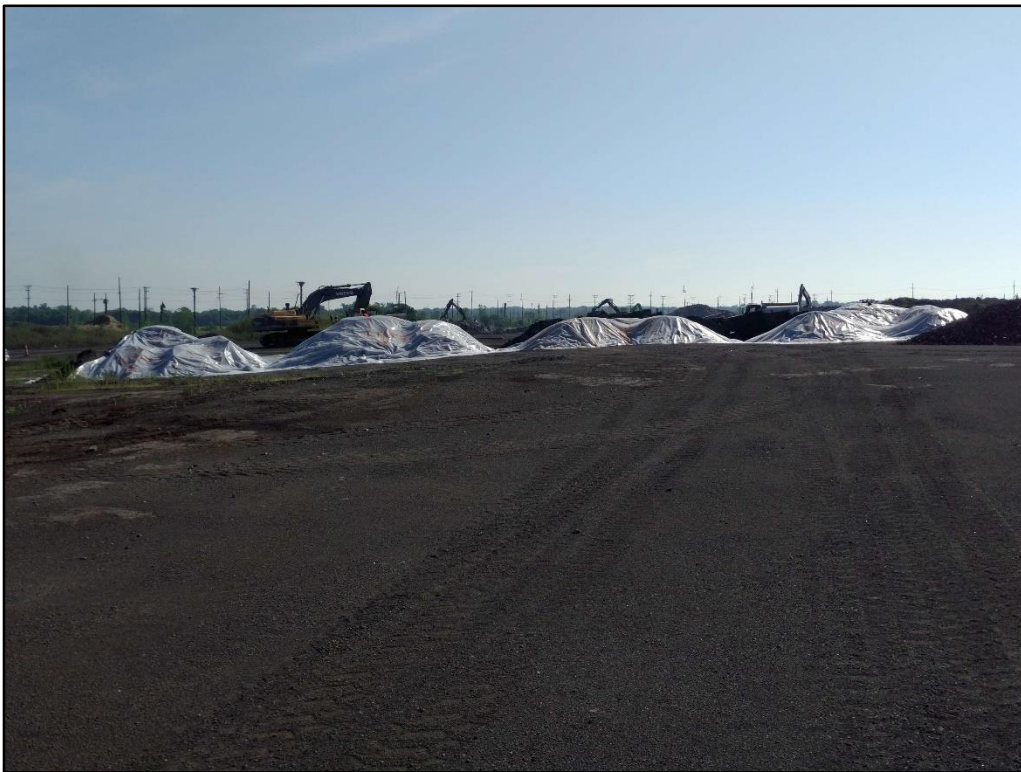
07/16/19-6: View to the east of the covered stockpiles.
