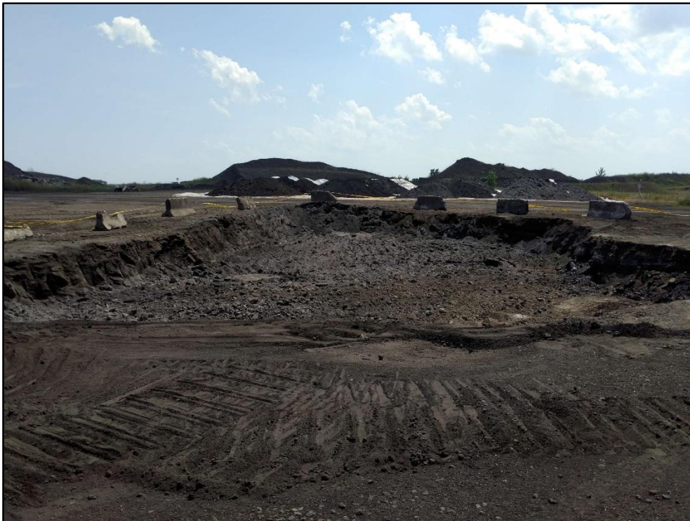
07/17/19-1: View to the west of the completed excavation.
