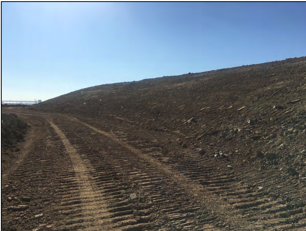
Photo 4: View of the exterior face of the eastern berm facing south.
