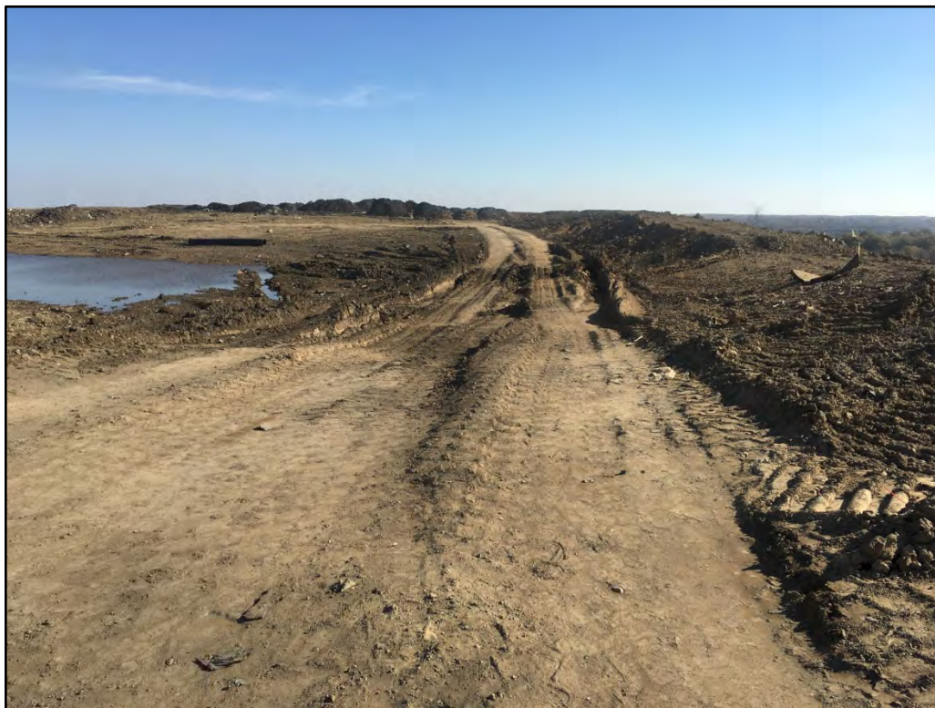
Photo 8: View of the interior face of the southern berm facing east.
