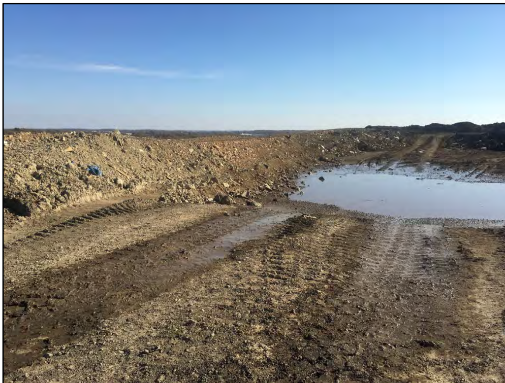
Photo 6: View of the interior face of the eastern berm facing east.
