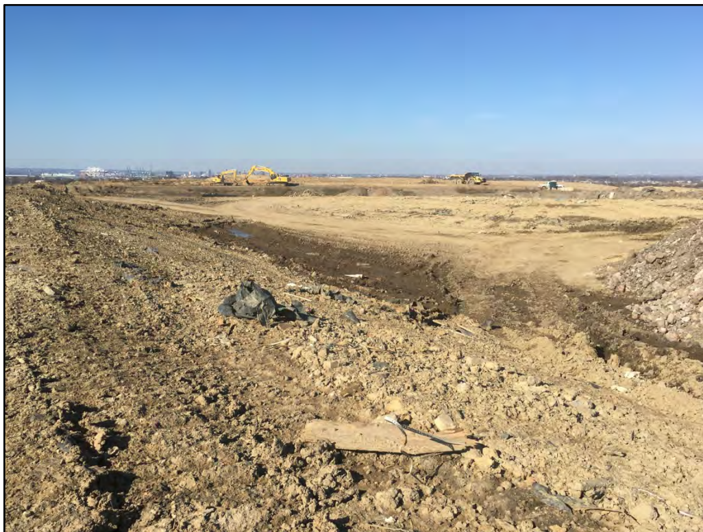
Photo 2: View of the cell facing west.
