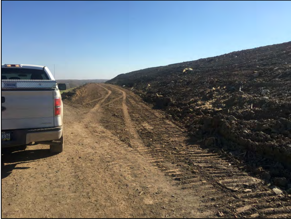
Photo 3: View of the exterior face of the northern berm facing east.
