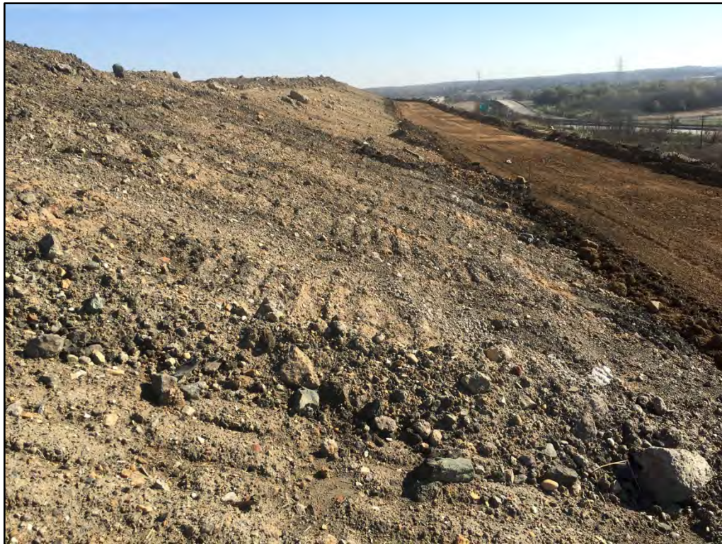
Photo 5: View of the exterior face of the southern berm facing east.
