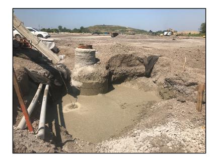
Photo 5: Trench plug construction
