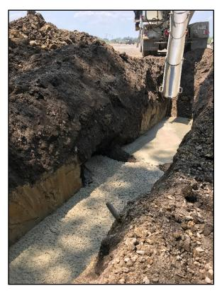
Photo 4: Trench plug construction
