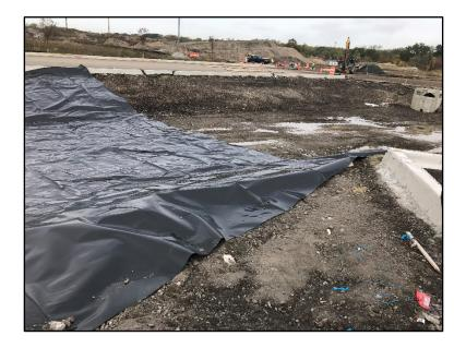
Photo 3: Installation of impermeable liner in stormwater basin
