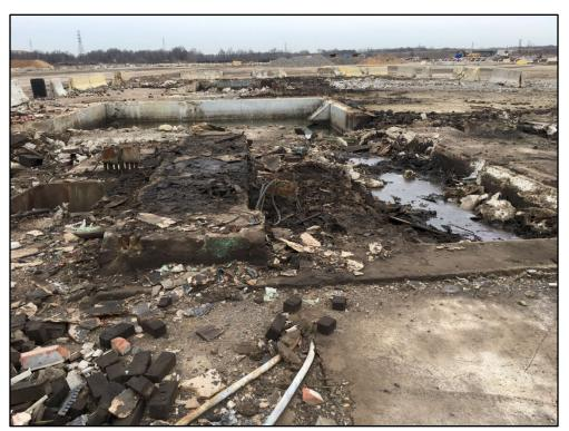
020118-4: Petroleum staining observed on the concrete of a shallow pit located on the northeastern portion of the parcel.
