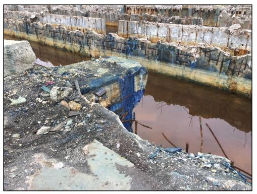
020118-8: Apparent sodium ferrocyanide (mixed with iron) impacts were observed along the concrete walls of the Halogen Line No. 1 and No. 2 located along the northern portion of the parcel. Halogen Line No. 2 can be seen in the background.
