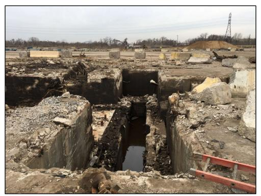
020118-6: Black colored NAPL observed on the water and petroleum staining on the concrete in a pit located towards the north-central portion of the parcel.
