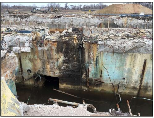
020118-7: Acid staining observed on the concrete in the eastern Halogen Line (No. 1) located on the northern portion of the parcel. Halogen Line No. 2 can be seen in the background.
