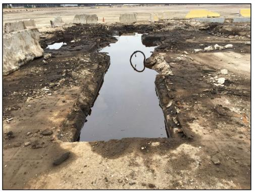
020118-3: Black colored NAPL observed on the water and petroleum staining on the concrete in a shallow pit located towards the middle portion of the parcel.
