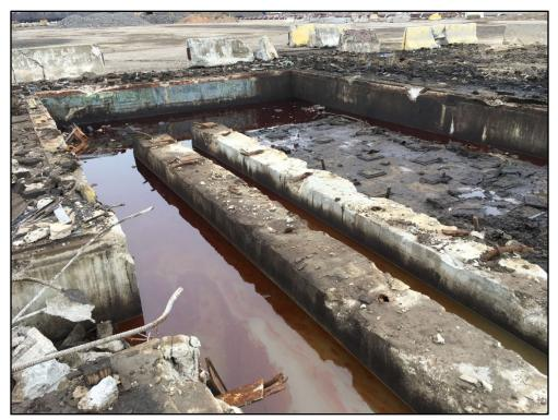
020118-2: Red colored NAPL observed on the water and petroleum staining on the concrete in a shallow pit located towards the middle portion of the parcel.
