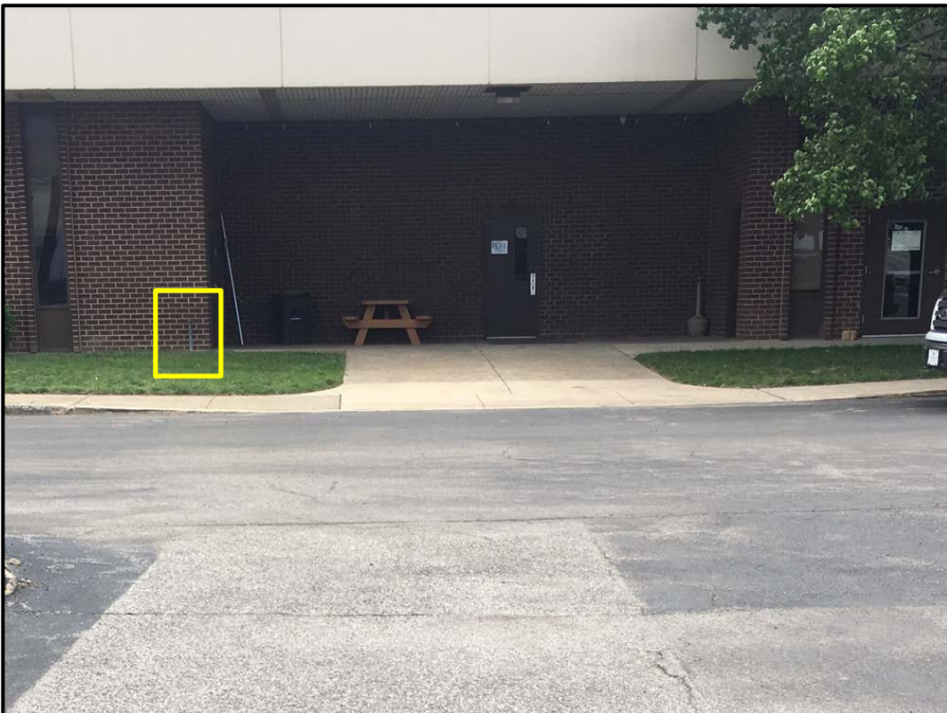
050317-2: Location of former Human Resources Building UST, facing east. Reference “vent pipe” is highlighted.
