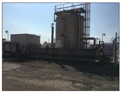
031518-13: View of an AST containing sodium hydrosulfide (NaSH) located south of the Tin Mill Canal along the parcel boundary line.
