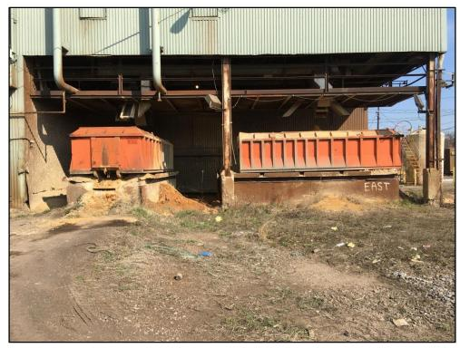
031518-15: View of the sludge bin filling area in which sludge filter cake from the wastewater treatment process enters the two sludge bins photographed above. These sludge bins are located under the Control Building.
