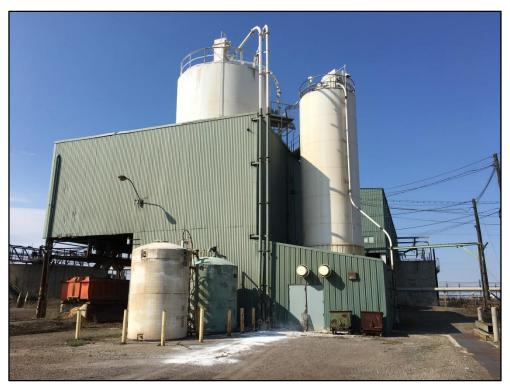
031518-14: View of additional ASTs and silos used to store unknown treatment chemicals as part of the wastewater treatment process located in and around the Control Building. The unknown white powder on the ground is presumed to be a water treatment chemical.
