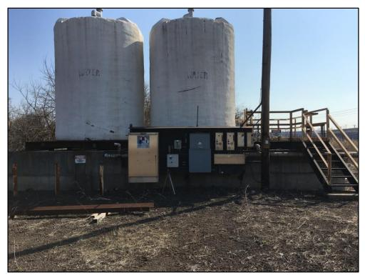
031518-12: View of two ASTs with secondary containment located north of the Tin Mill Canal. The ASTs are labeled "WATER" but the danger sign states "CAUSTIC" and the hazardous material placard also indicates caustic.
