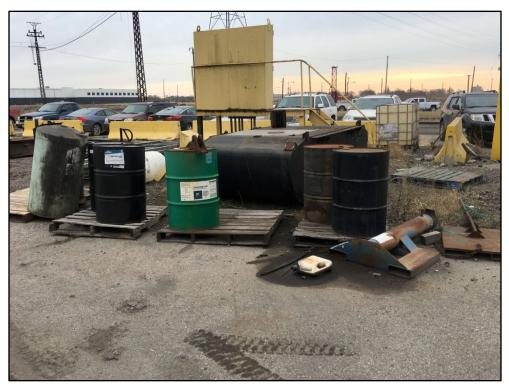
020118-12: Miscellaneous temporary storage of several drums/tanks outside of the Locomotive Shop to the east. Staining observed on ground surface.
