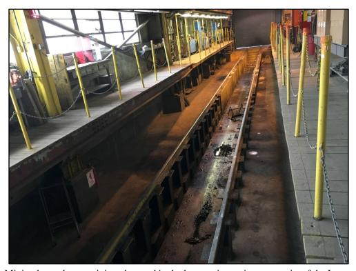
020118-8: Minimal petroleum staining observed in the locomotive maintenance pits of the Locomotive Shop.
