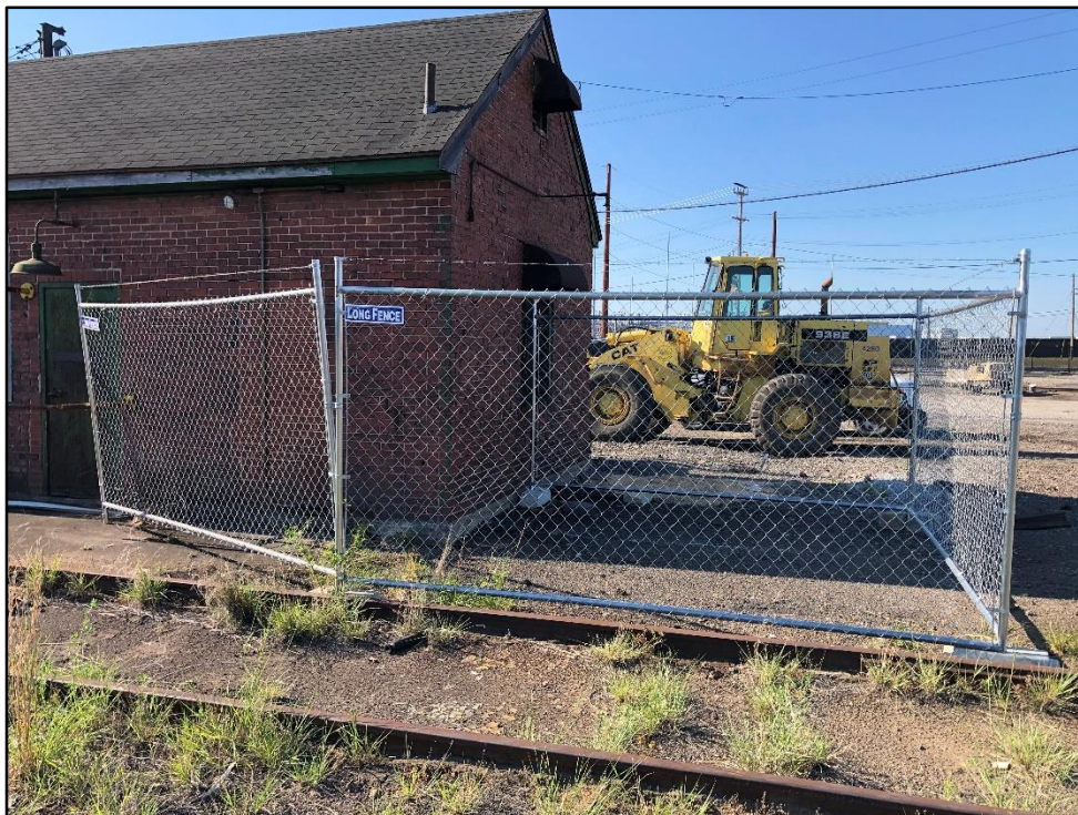
062920-2: Temporary fencing installed around boring B23-010-SB.
