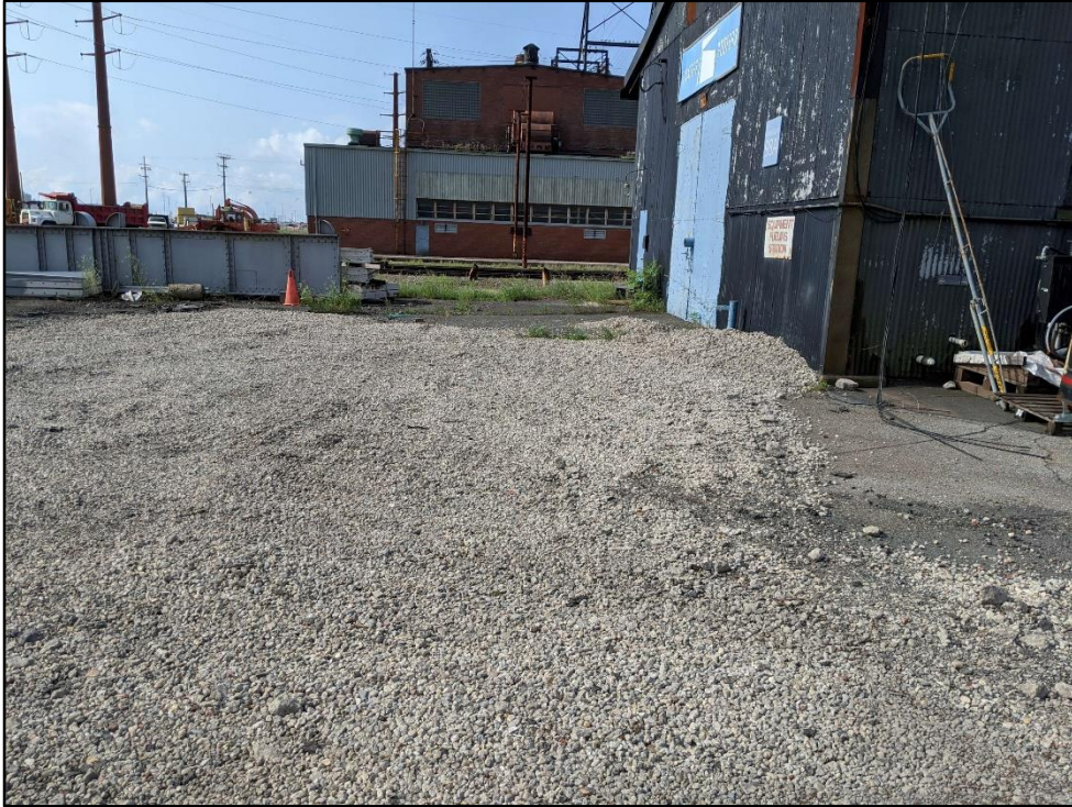
070820-4: Crushed recycled concrete temporary cap installed covering boring B23-034-SB.
