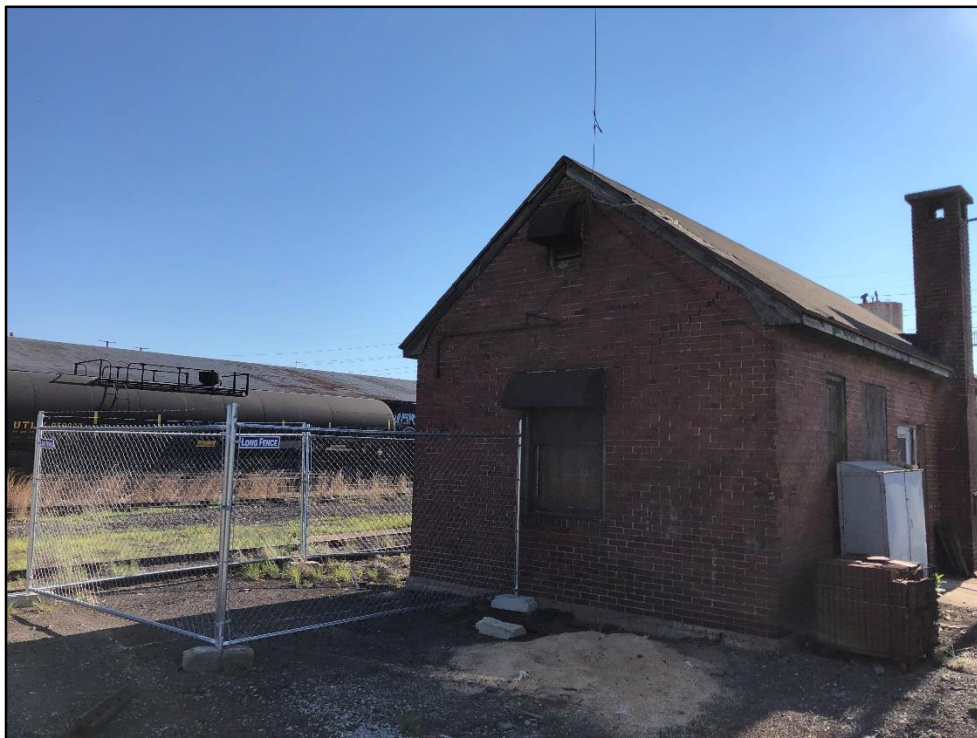
062920-1: Temporary fencing installed around boring B23-010-SB.
