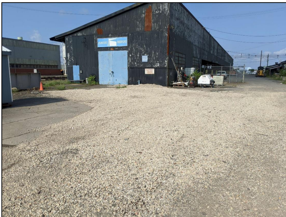
070820-3: Crushed recycled concrete temporary cap installed covering boring B23-034-SB.
