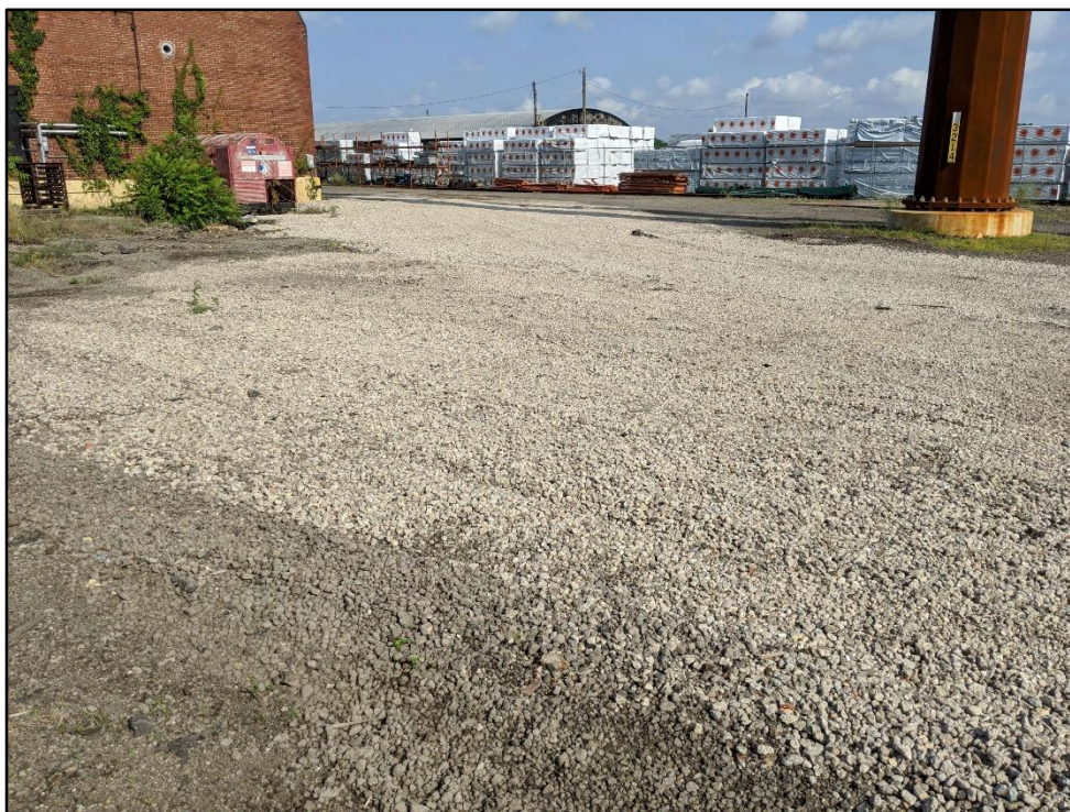
070820-1: Crushed recycled concrete temporary cap installed covering boring B23-016-SB.
