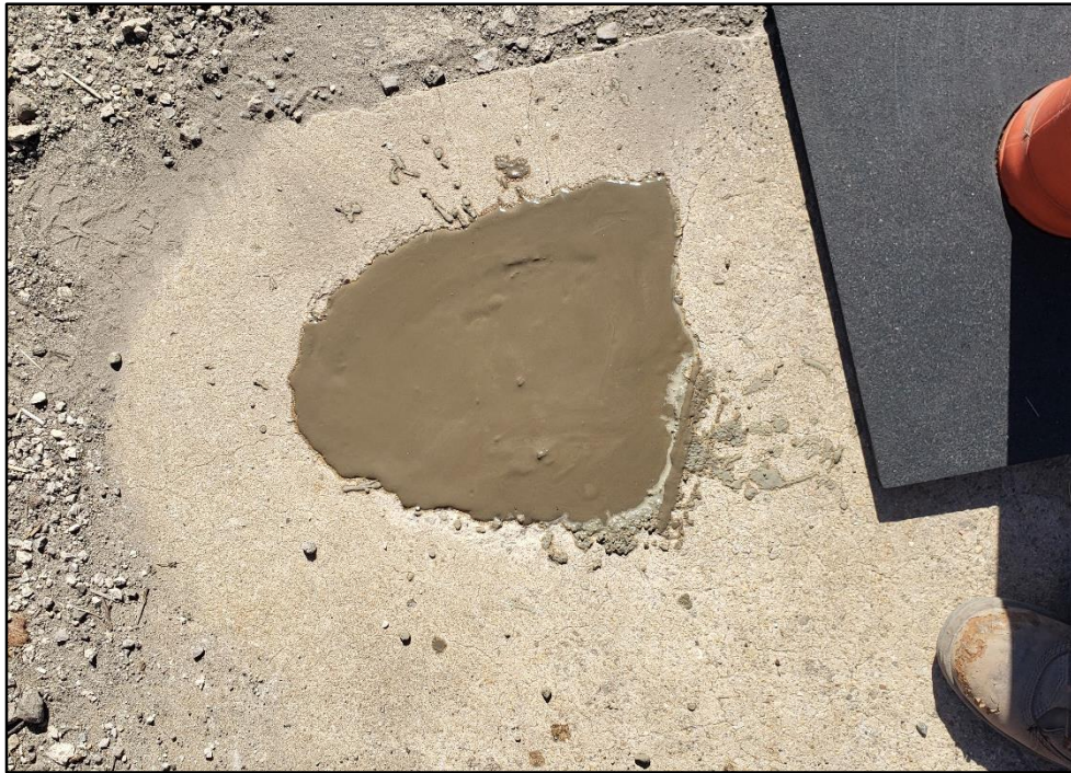
060820-1: Concrete patch installed at boring hole for B23-015-SB.
