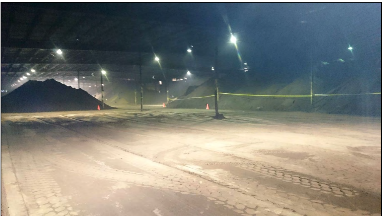
083116-8: Open area in the northwest corner of the warehouse, facing southeast. Stockpiles in background.
