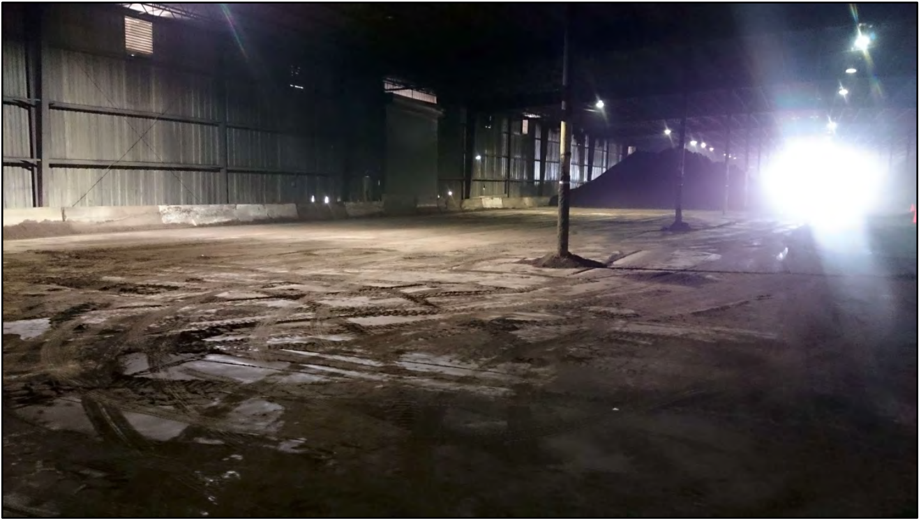
083116-7: Open area in the northwest corner of the warehouse, facing northeast. Open bay doors (east) visible.
