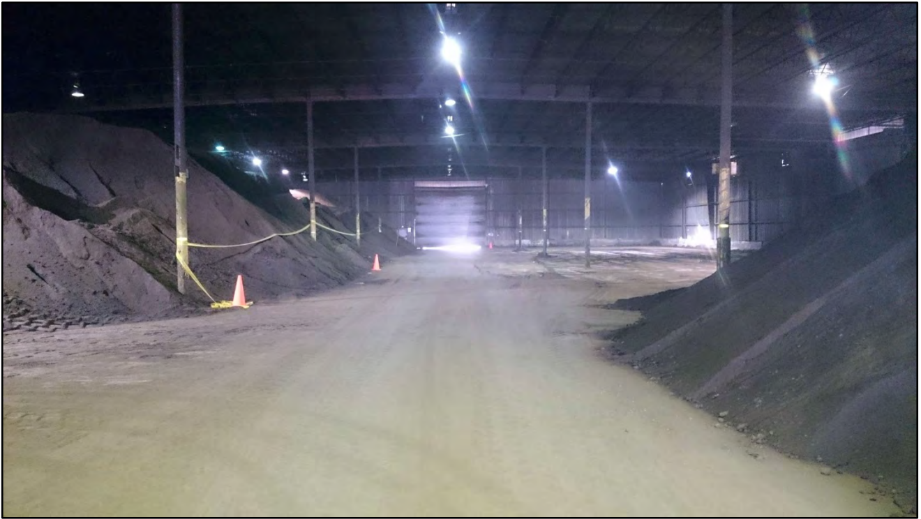
083116-5: Western half of warehouse with open bay doors in background, facing west. Stockpiles and open areas visible.
