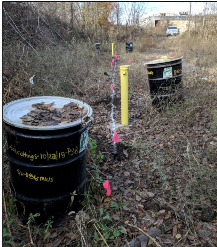
Photo 6: Field confirmed alignment of sheet piling, following well installation (facing north).
