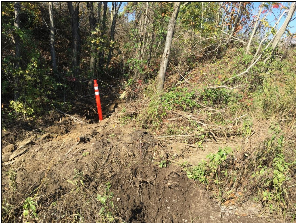
Photo 2: Northern extent of the sheet piling.
