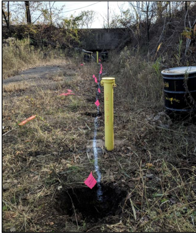
Photo 5: Field confirmed alignment of sheet piling, following well installation (facing south).
