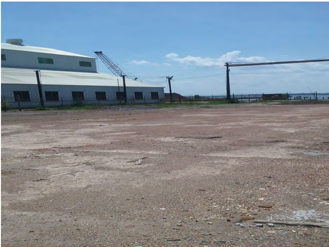
060116-4: Southwest corner, facing southwest.
