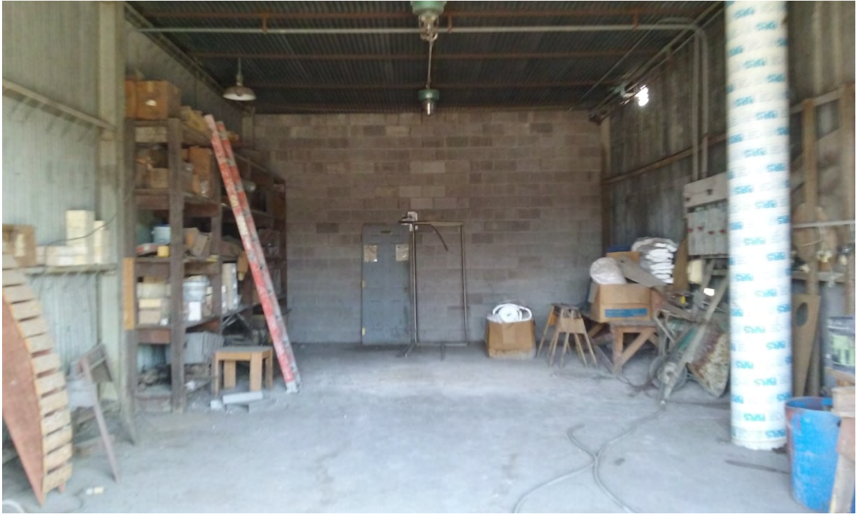
082616-1: Most eastern room (of five rooms) in the enclosed section of the south Brick Shed. Picture facing north.
