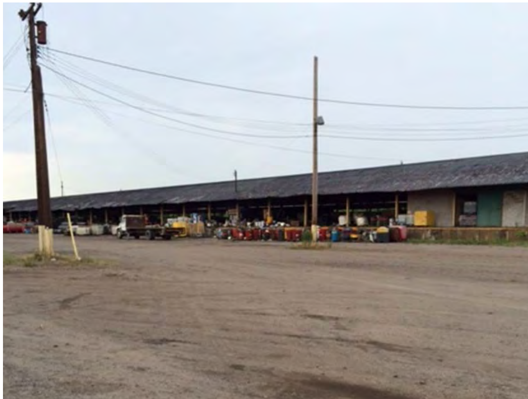
061516-2: Northeastern corner of the parcel with existing buildings (brick sheds), facing northwest.
