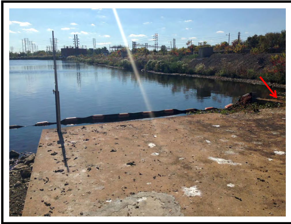
Photo 5: Looking south from concrete platform. Discharge pipe and culvert are to the west.
