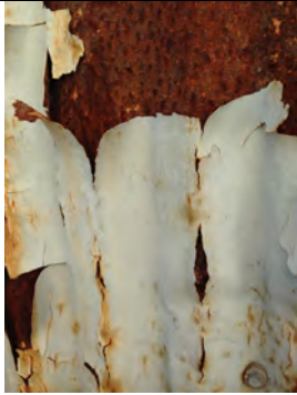
Photo 8: Sheet Metal Siding Paint Exterior Walls/Roof
