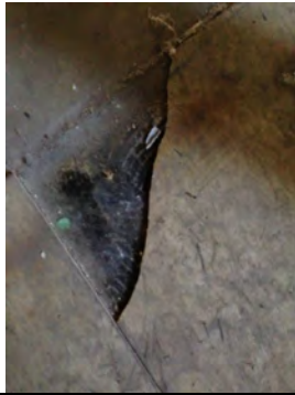
Photo 6: 12x12 Off White Floor Tile w/Black Mastic
