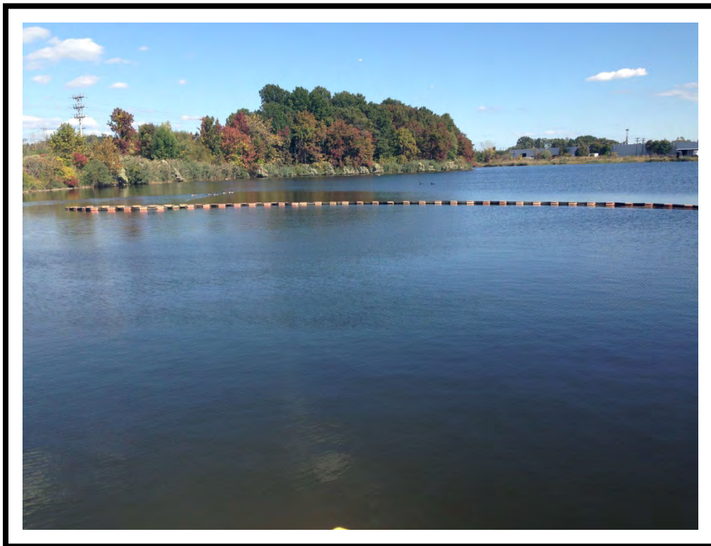
Photo 6: Looking northeast from concrete platform at baffle (boom) on High Head Reservoir.
