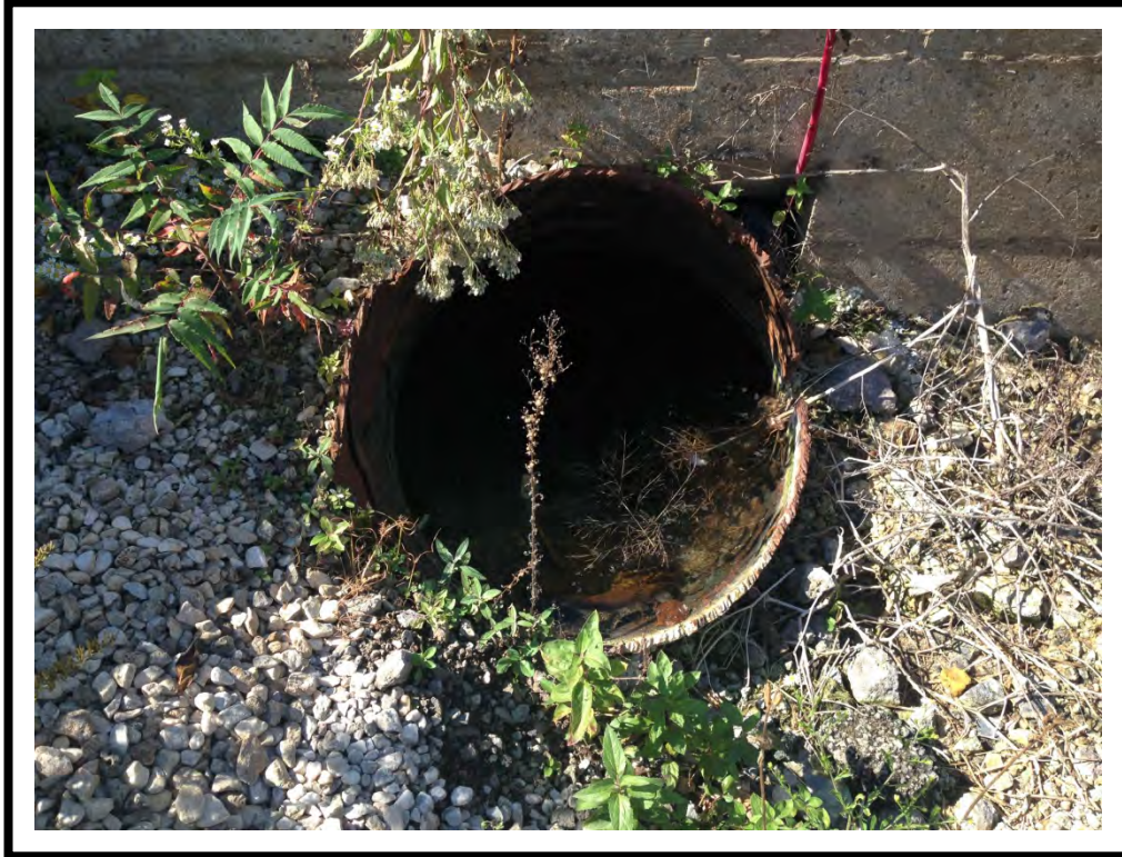
Photo 1: Outfall/drain pipe in REC 11B area.
