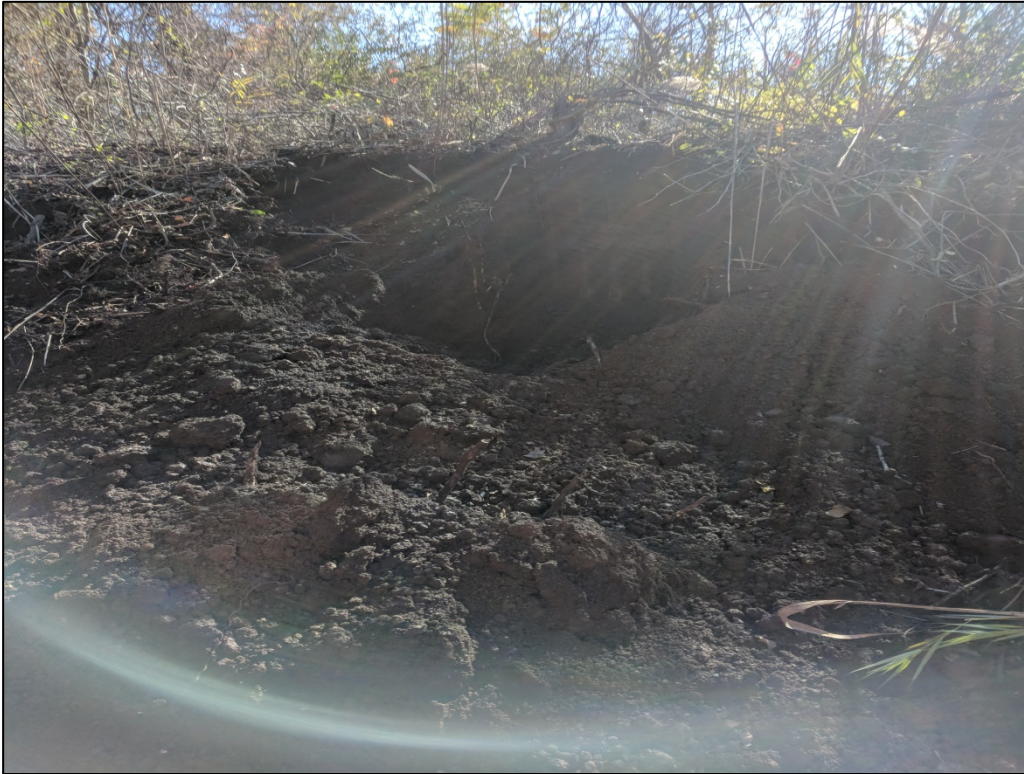
Photo 27: View of test pit at A7-010-TP after excavation. No visible contamination is evident and PID reading equals 5.4.
