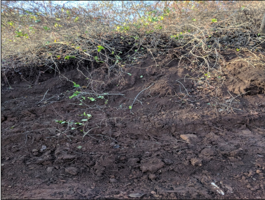
Photo 1: View of test pit at A7-001-TP before excavation. No visible contamination is evident.
