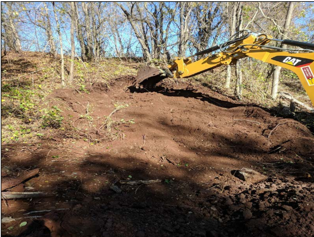
Photo 18: View of test pit at A7-007-TP before excavation. No visible contamination is evident.
