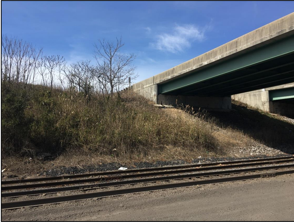
032819-1: View of highway overpass at the northern border of the Site.
