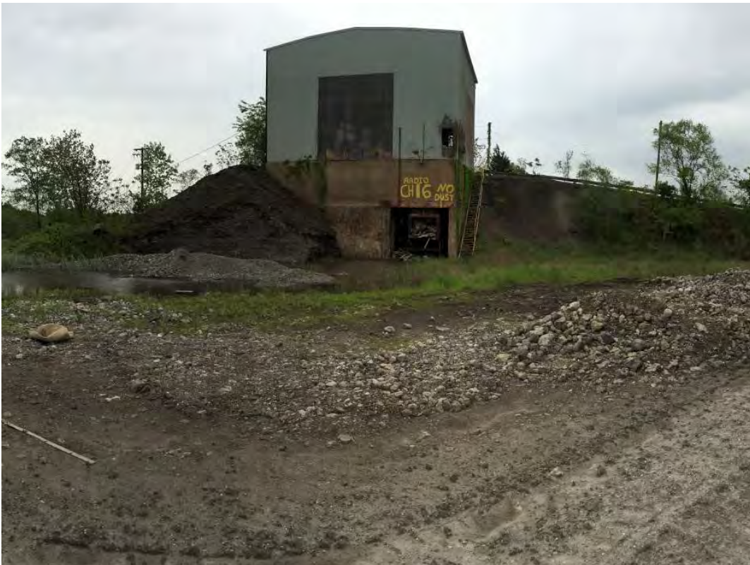
050916-8: Trash transfer station from roadway in spare parts yard, facing southwest.
