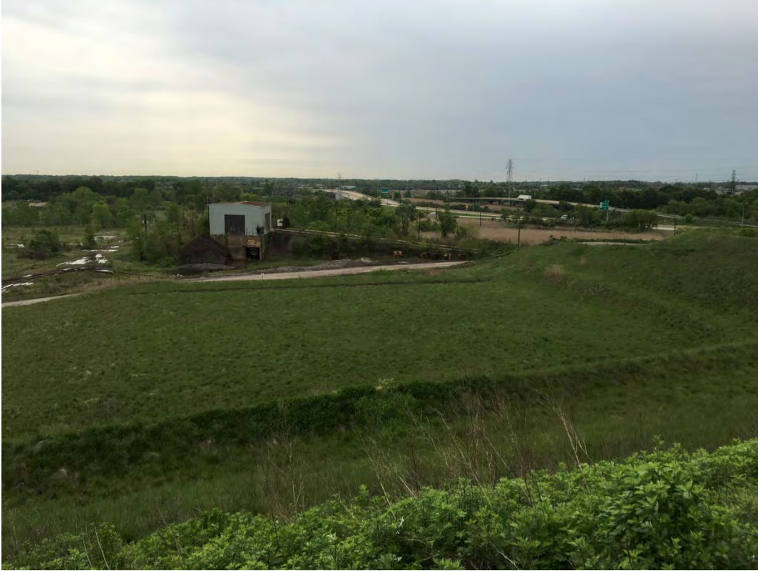
050916-7: Trash transfer station (from top of Greys Landfill), facing southeast.
