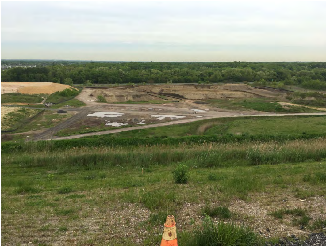
050916-3: Former spare parts yard occupied by soil stockpiles (from top of Greys Landfill), facing northeast.
