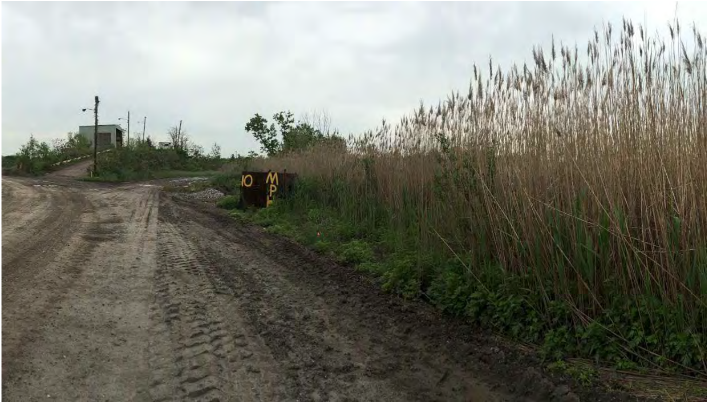
050916-9: Trash transfer station from roadway at the base of Greys Landfill, facing northeast.
