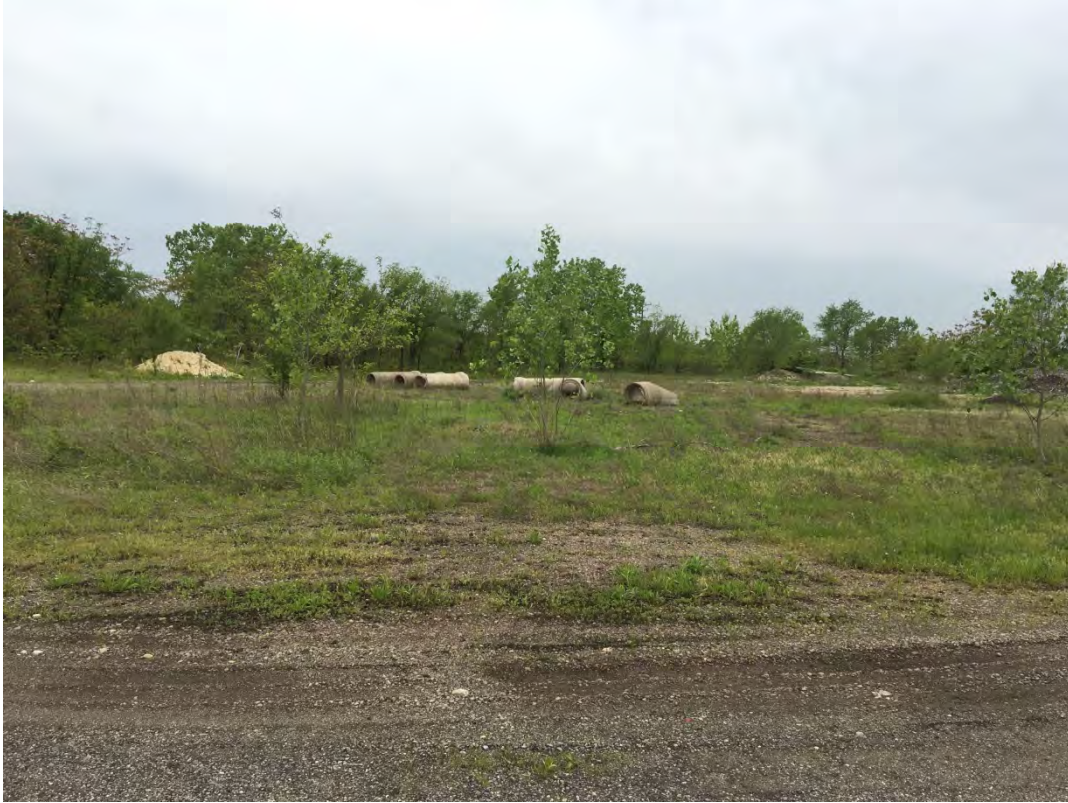
050916-13: Contractor area largely vacant with some loose debris piles, facing south.
