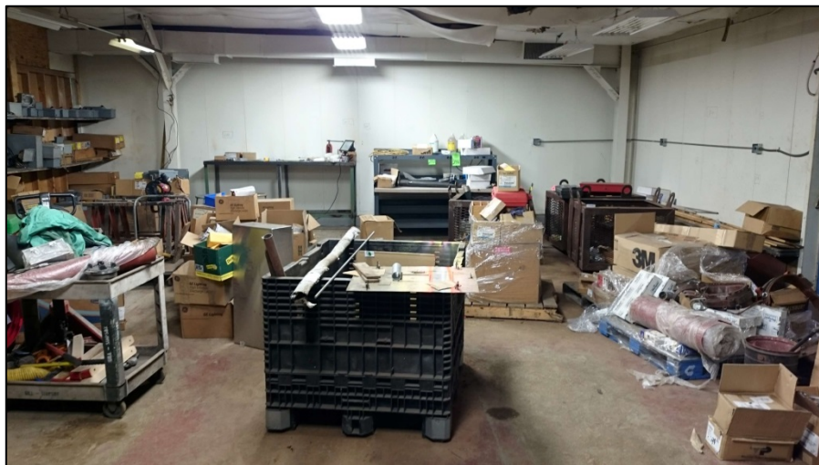
030216-3: Storeroom & Shop. Main room with generic storage (primarily electrical equipment), facing southeast.
