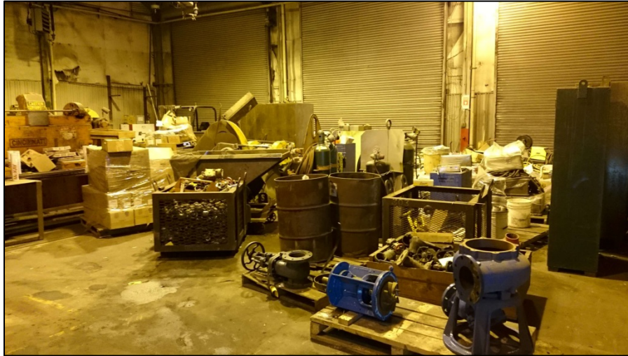
030216-19: Repair Shop. Interior view of bay doors and generic storage, facing northwest. No hazardous materials noted.
