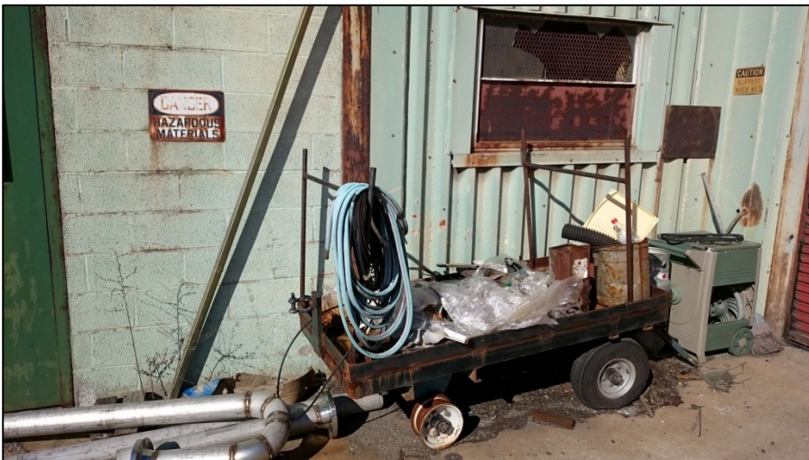
030216-14: Repair Shop. Exterior view with hazardous label, facing west. Former location of PVC glue spill.
