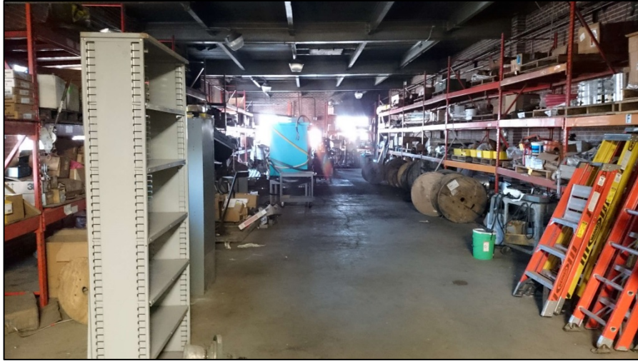
030216-4: : Storeroom & Shop. Main room with generic storage (primarily electrical equipment), facing northwest.
