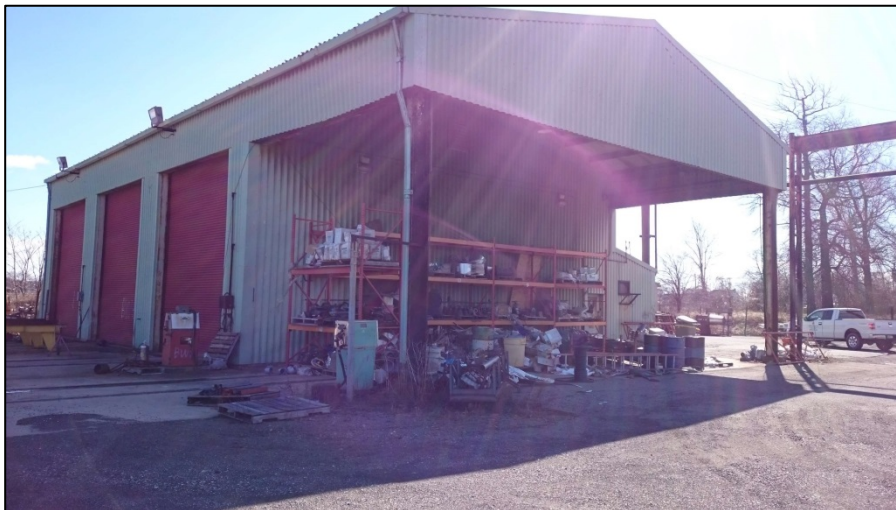
030216-11: Repair Shop. Exterior view of shop building, facing southeast.
