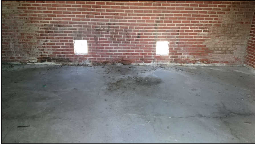
030216-1: Oil House. Interior view of vacant building, facing southwest.
