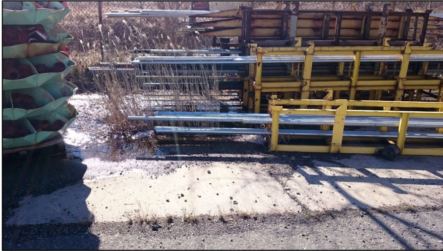
030216-16: Repair Shop. View of concrete pad located southeast of main shop, facing south. Possible fuel UST location.
