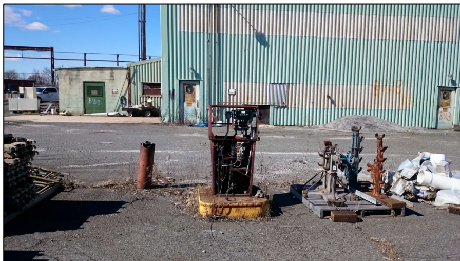
030216-12: Repair Shop. Exterior view of shop building, facing west. Noted location of fuel pump.
