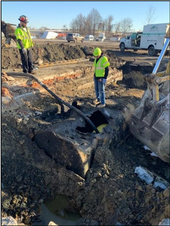
020320-1: ACE Environmental personnel removing remaining UST contents using a vacuum truck.
