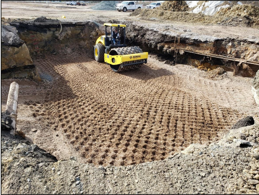
022420-1: Backfilling and rolling a lift of the excavation.
