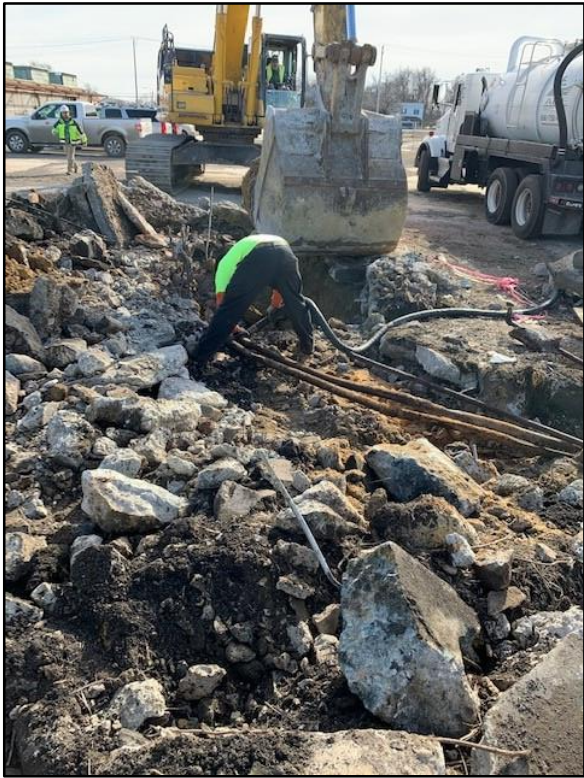
020320-5: Removal of pipes revealed during excavation and UST removal.
