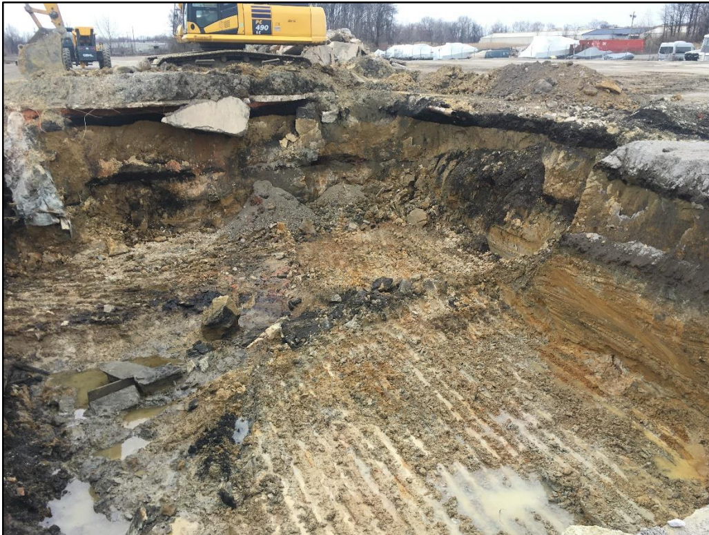
022020-2: Eastern test pit excavation
