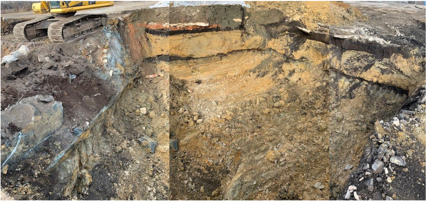
020520-2: Panorama view of eastern test pit excavation.
