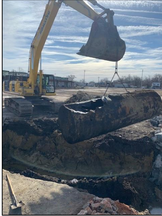
020320-2: Removal of the uncovered empty UST using the excavator.
