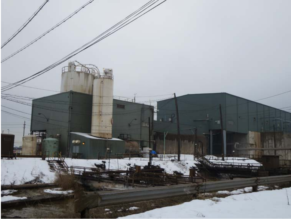
Photo 15: View of the Humphrey Creek Wastewater Treatment Plant.
