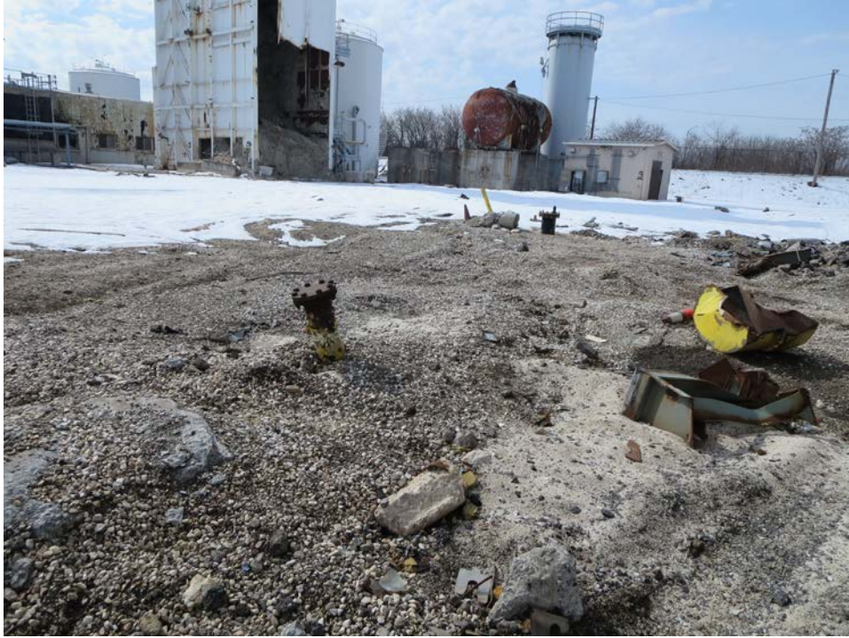
Photo 3: View of the Air Products Facility debris and SACM.
