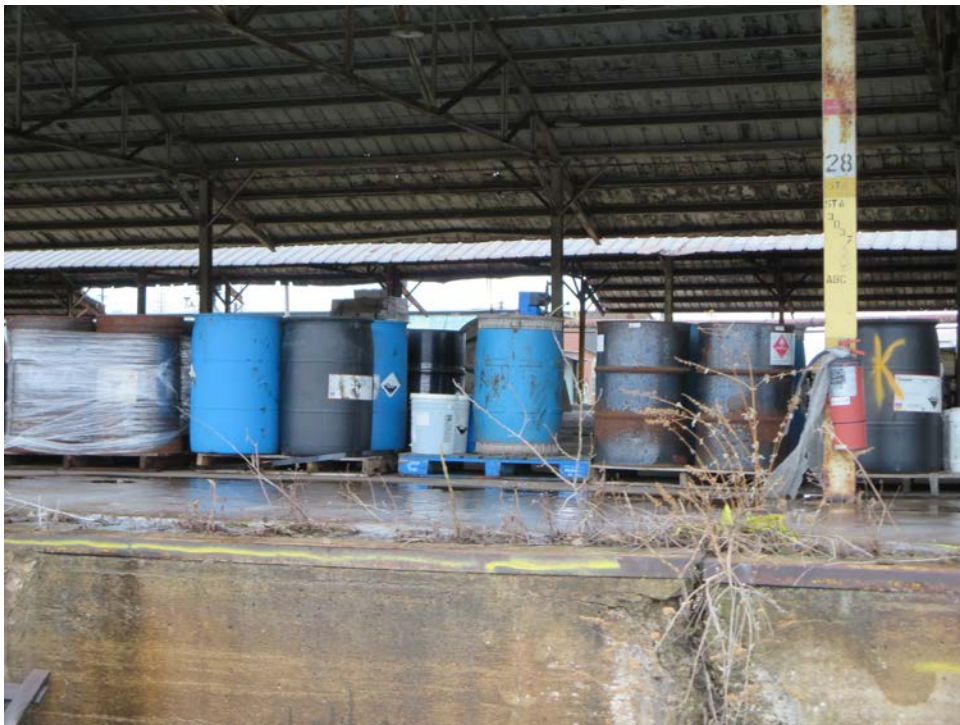
Photo 14: View of the brick chemical storage building.
