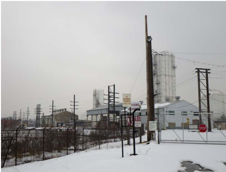
Photo 2: View of the Air Products Facility.
