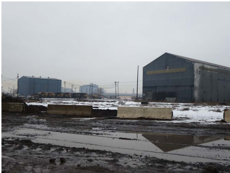
Photo 40: General view of the Coke Oven area.
