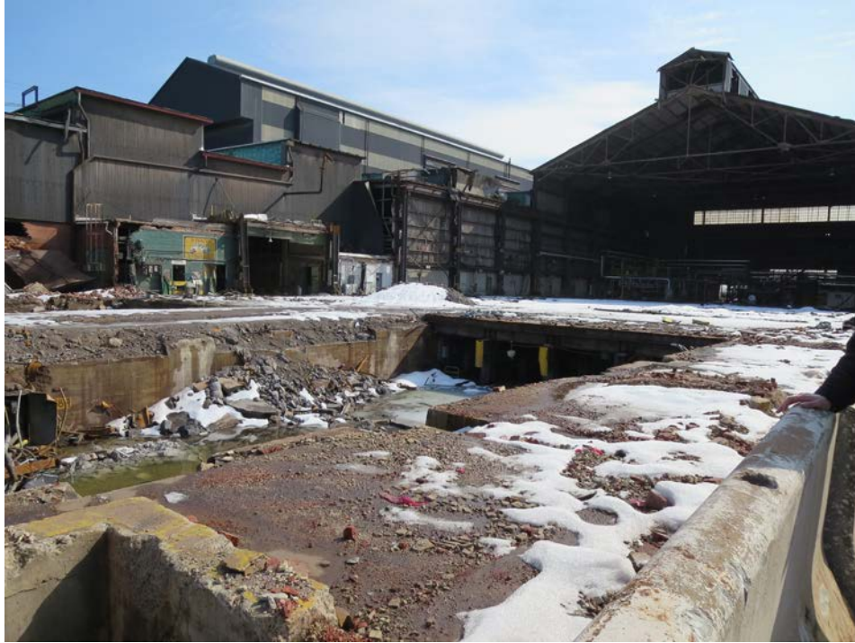
Photo 21: View of the old Cold Mill demolition.
