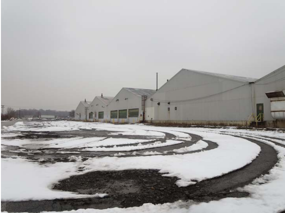
Photo 1: View of the reservoir warehouses.
