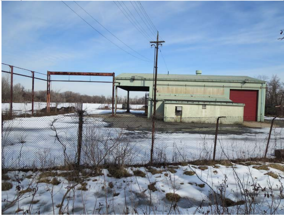
Photo 5: View of the Maintenance of Way Yard.
