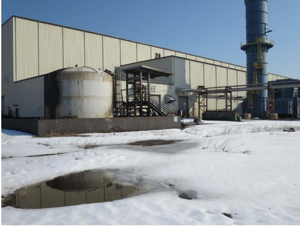
Photo 9: View of the new Cold Mill building.
