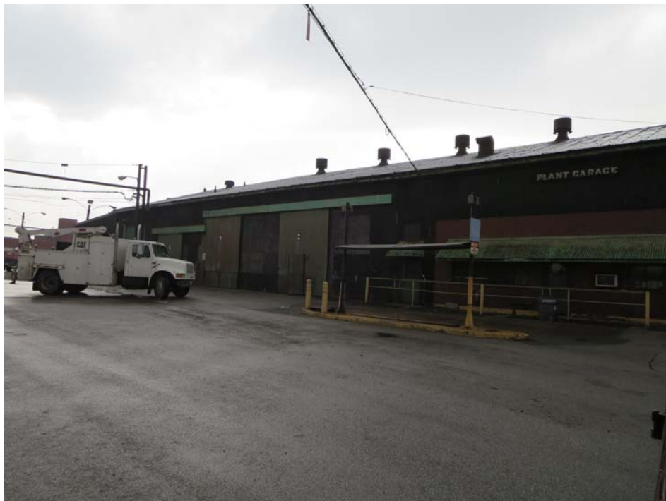
Photo 28: View of the plant garage.
