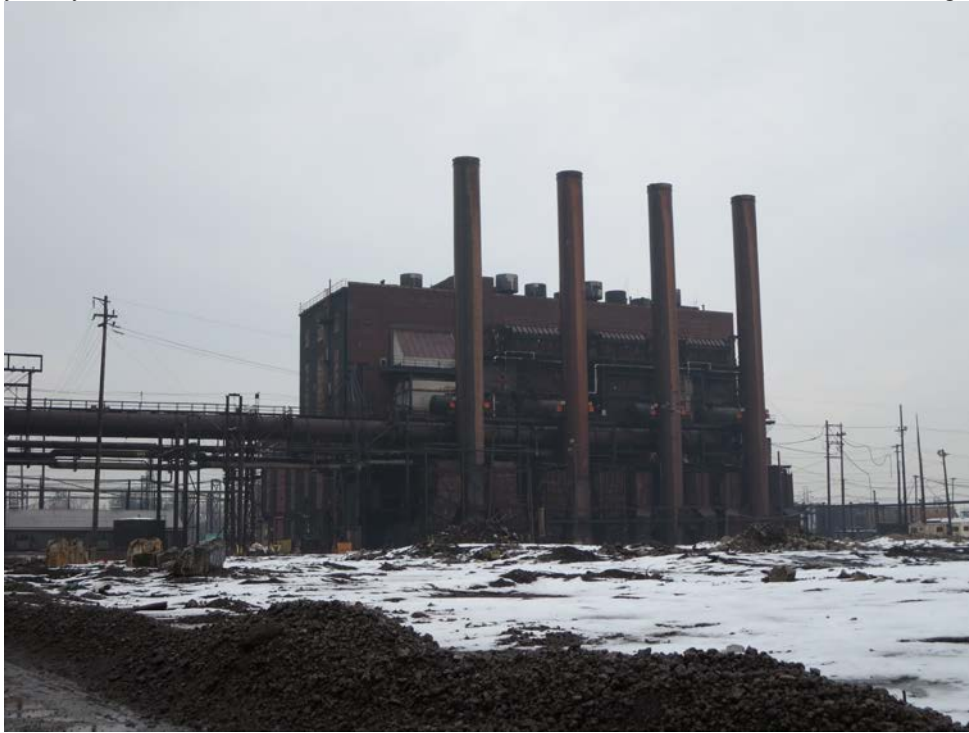
Photo 31: View of the Penwood Powerhouse.
