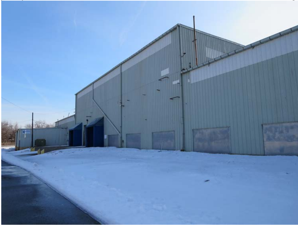
Photo 47: View of the Dietrich building.
