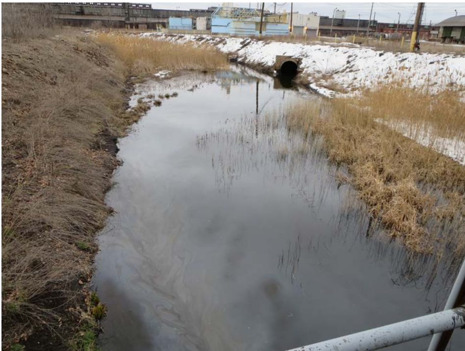
Photo 12: View of the Tin Mill Canal.
