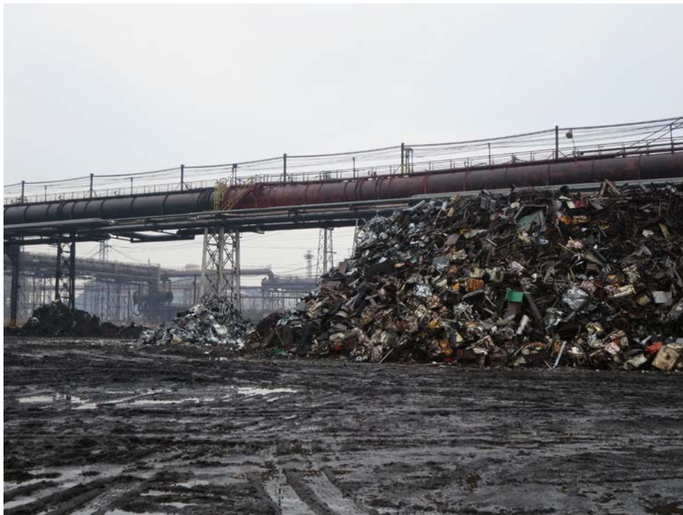
Photo 34: Representative view of the demolition debris piles.
