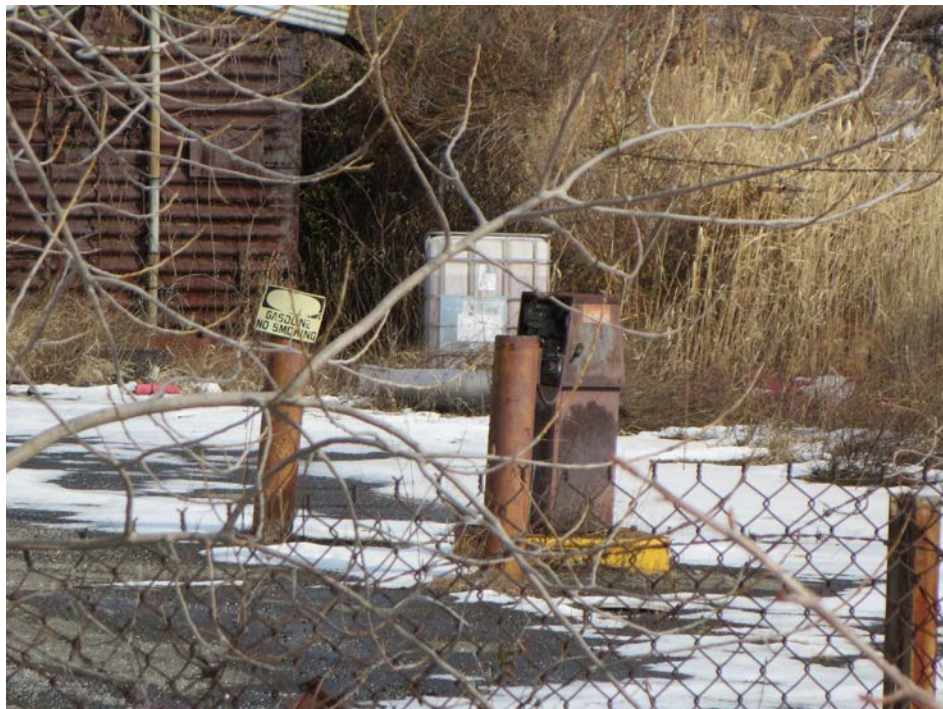
Photo 6: View of the Maintenance of Way Yard filling station.
