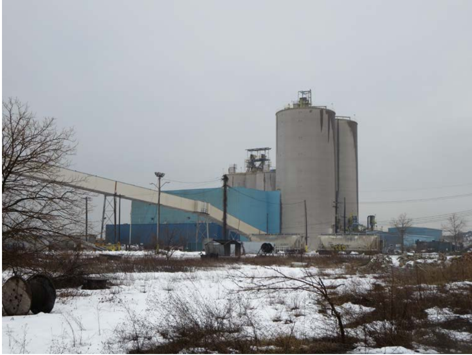
Photo 43: View of the Lafarge building.
