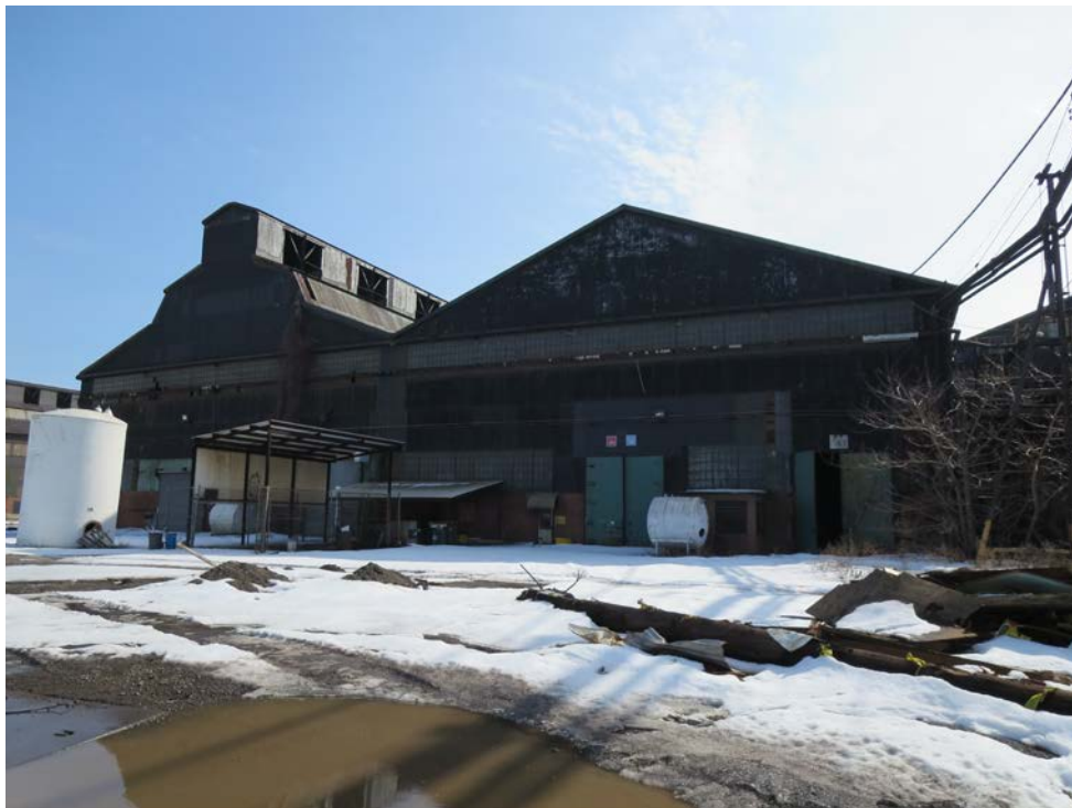
Photo 20: View of the old Cold Mill and tank/drum storage.
