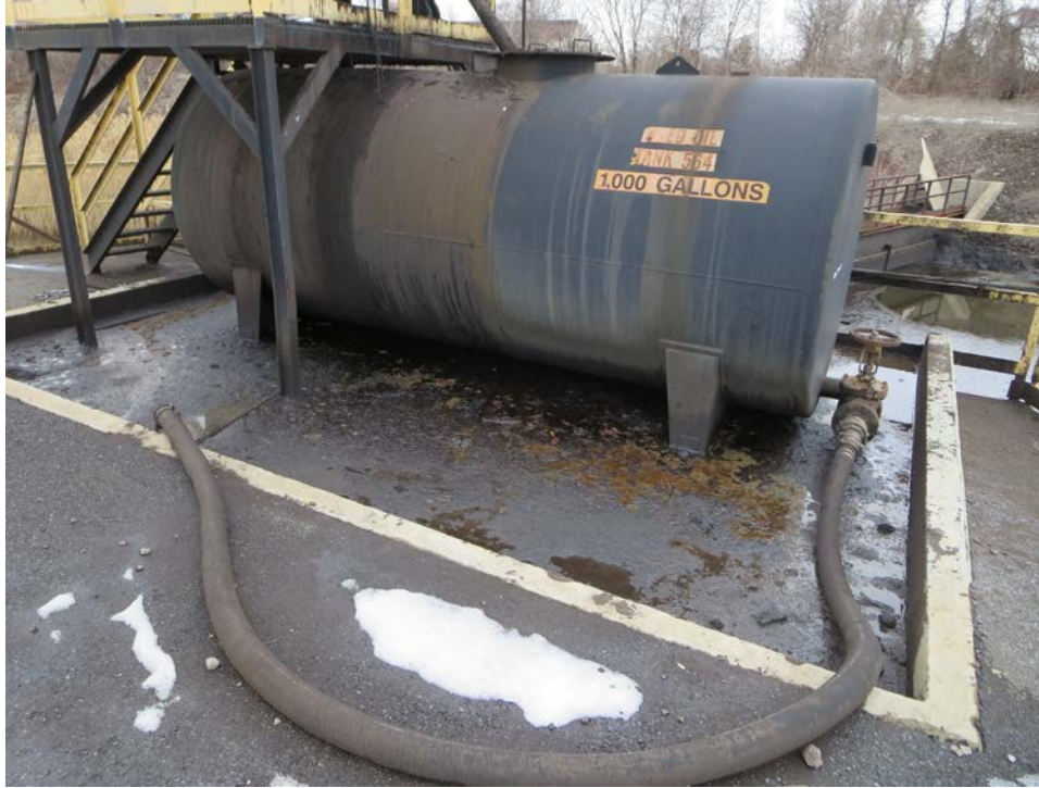
Photo 13: View of used oil AST and leaking into the Tin Mill Canal.
