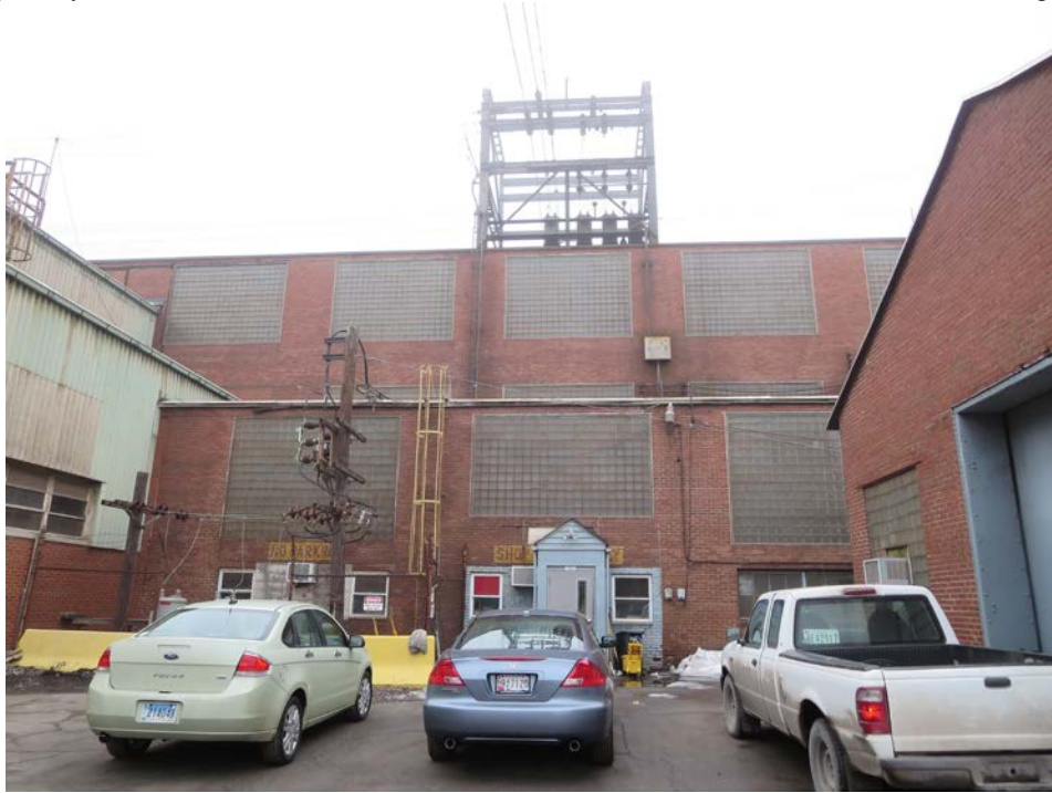
Photo 25: View of the railroad shop building exterior.
