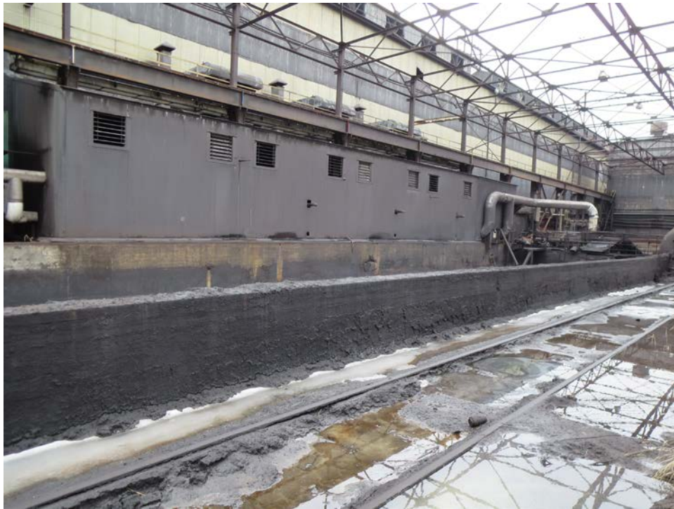
Photo 16: View of the Hot Strip Mill scale pit.
