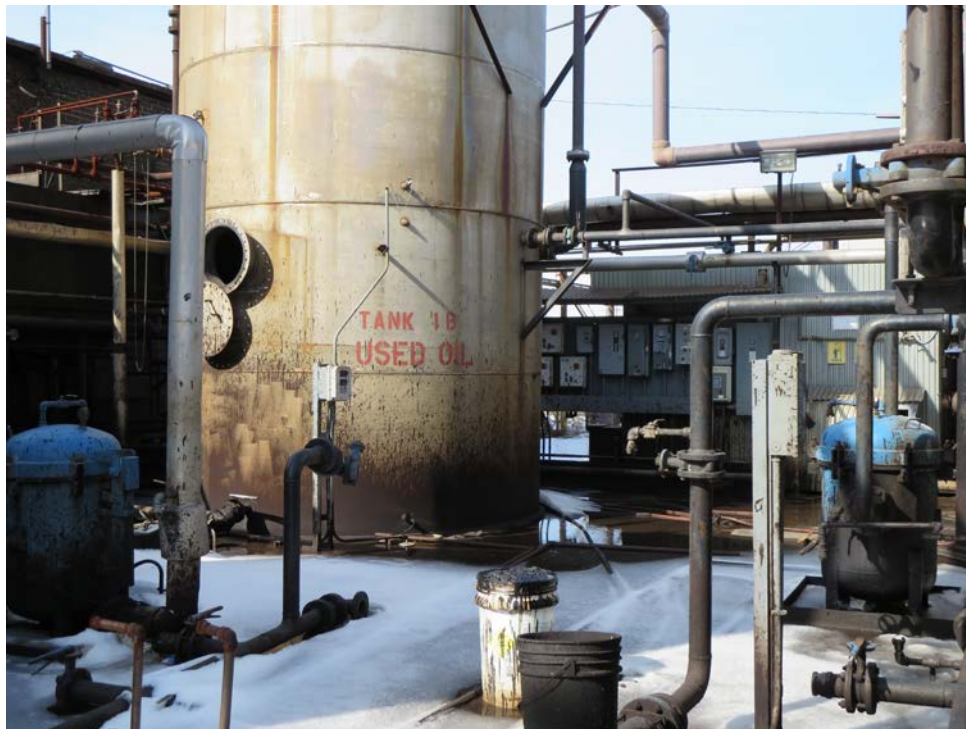
Photo 22: View of tanks north of the Tin Mill.
