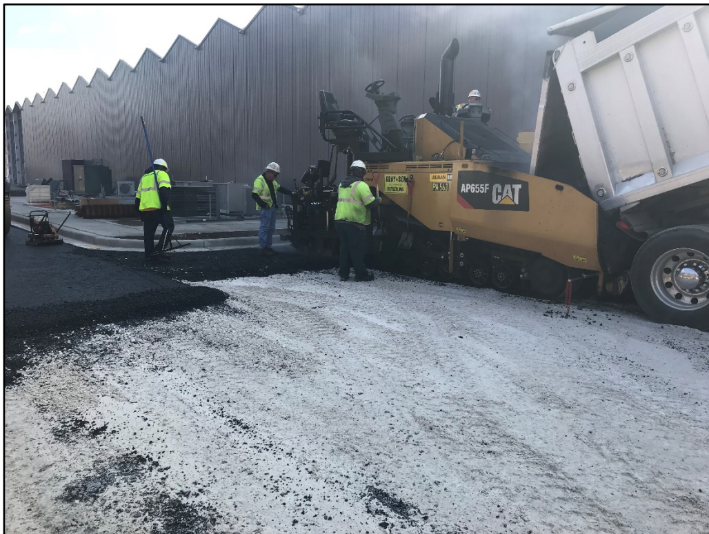
Photo 6: Surface paving
