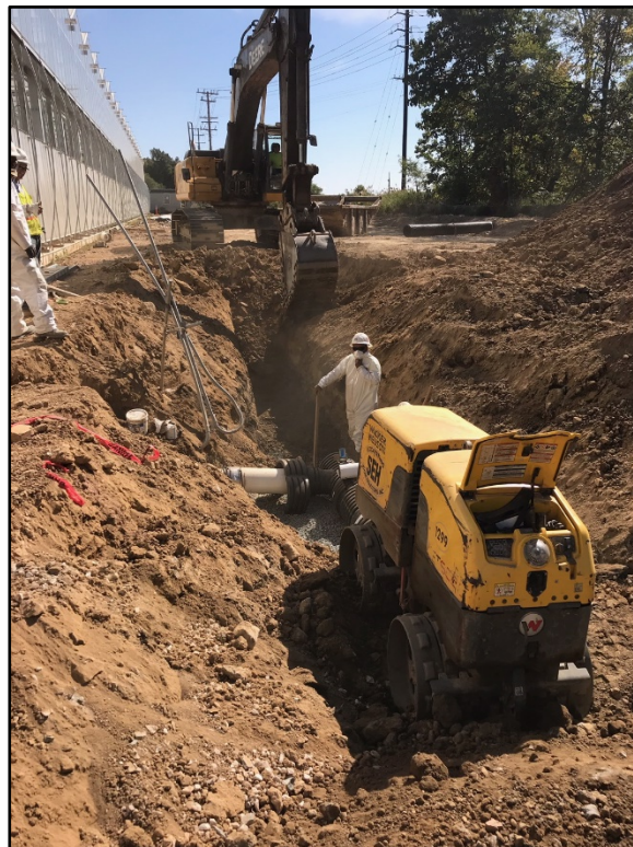
Photo 4: Utility excavation and installation
