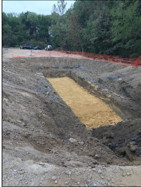
Photo 5: Utility excavation backfilling
