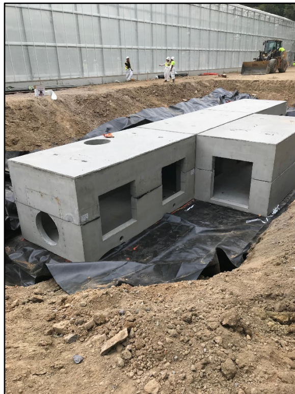
Photo 2: Utility installation
