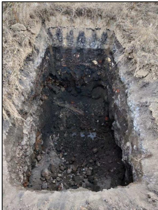
100419-2: View to the northeast of the completed southern excavation.
