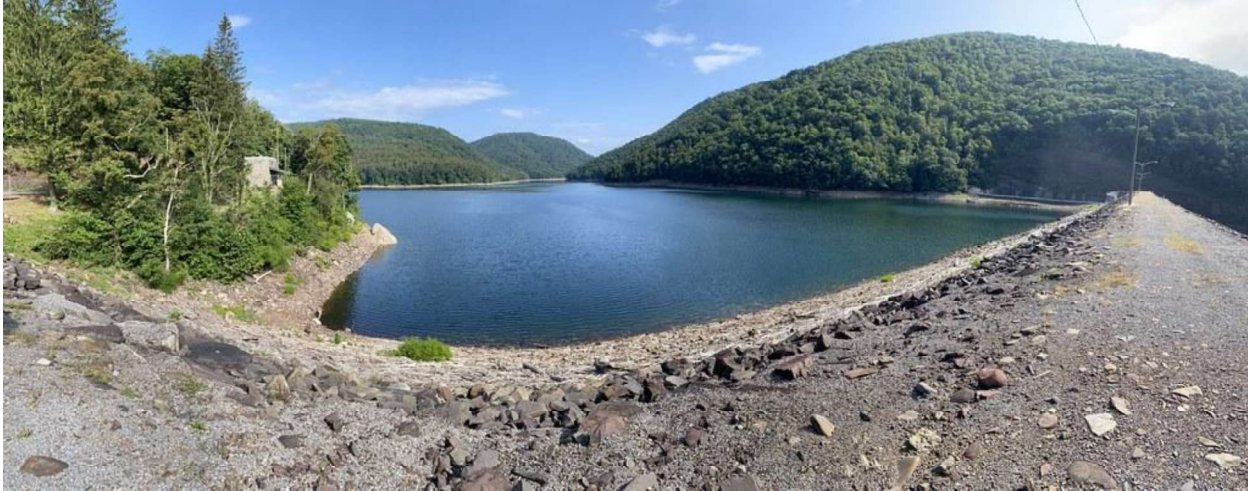
Savage River Dam, Garrett County Maryland
