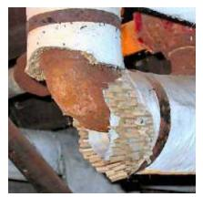
Damaged asbestos pipe insulation
