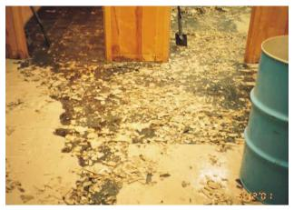
**Photo** #7 - The floor tile was removed using an ice chipper and is friable. Floor tile being removed in this manner must be removed according to the MDH Asbestos Abatement Rules.
