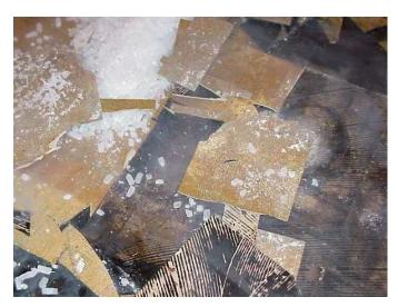
**Photos #5 & #6** - The floor tile in these photos are friable. It was removed with the hand tools that can be seen near the top of Photo #6. Floor tile being removed in this manner must be removed according to the MDH Asbestos Abatement Rules.
