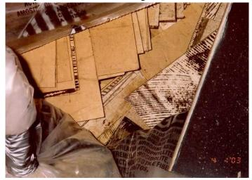
**Photos #3 & #4** - The asbestos-containing floor tile in these photos was removed with dry ice and an ice chipper. Too much breakage is occurring to the floor tile. If the project continues in this manner, it is considered a regulated project, subject to all MDH asbestos regulations. MDH recommends stopping the current removal method and changing to a method that reduces breakage.
