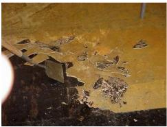
**Photo** #8 - The floor tile in this picture may have been removed nonfriably and then placed in a lined fiber drum. The work crew used a hand tool to break up the floor tile in order to fit more into the drum. The floor tile has now become friable during the handling process. The floor tile needs to remain nonfriable from removal until it is disposed of.
