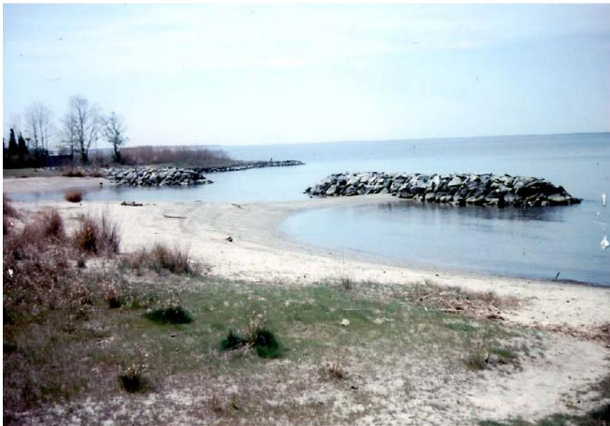
**Fig. 34. Large offshore breakwaters, with opening.** (Photo: Maryland Department of Natural Resources)
