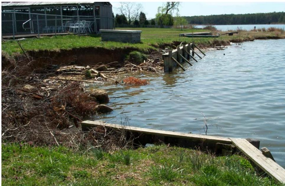
**Fig. 32. Catastrophic bulkhead failure, resulting in need to replace entire structure with different stabilization practice.** (Photo: Maryland Department of the Environment)
