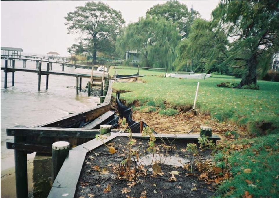
**Fig. 31. Failed bulkhead with erosion behind structure.** (Photo: Maryland Department of Natural Resources)
