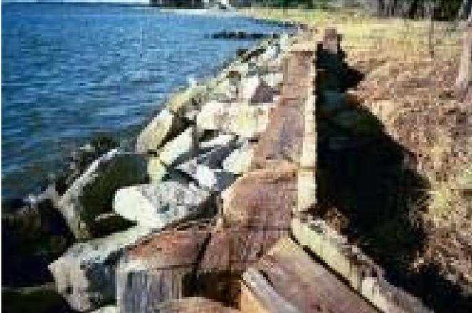
**Fig. 30. Collapsing bulkhead with additional riprap.** (Photo: Maryland Department of Natural Resources)
