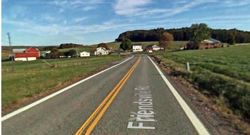
Figure 4. Friendsville 1, near the location of the traffic counter south of the Pennsylvania border (Google Maps).
