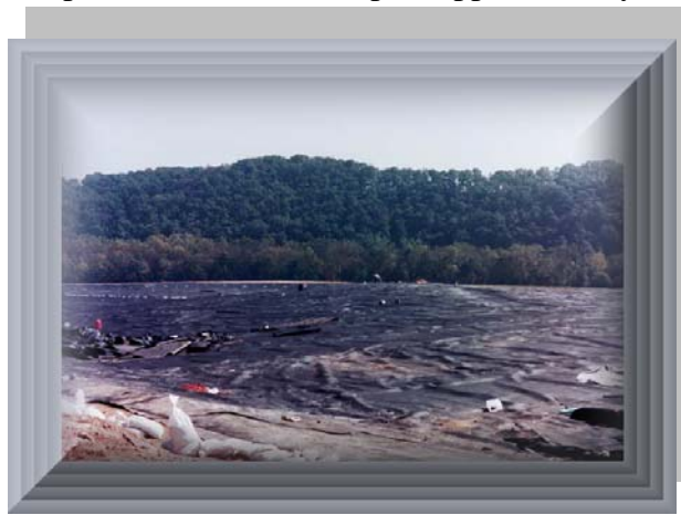
Landfill Liner Installation.
