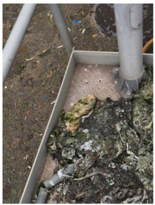
3/22/22 Scum collected from center well is not being disposed of properly
