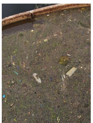
3/22/22 Center well of clarifier filled with floating debris
