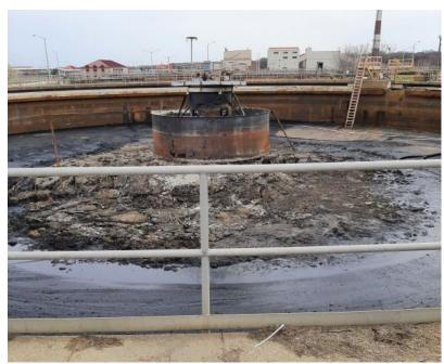
Inactive PST due to solids buildup 3/22/22
