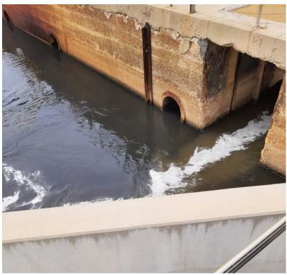
3/22/22 wastewater from PSTs going to the biological reactors Ferric chloride is added to the waste stream at this point
