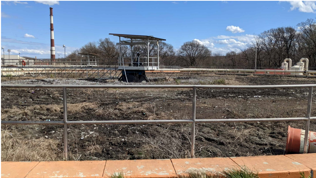
Primary Sedimentation Tank
