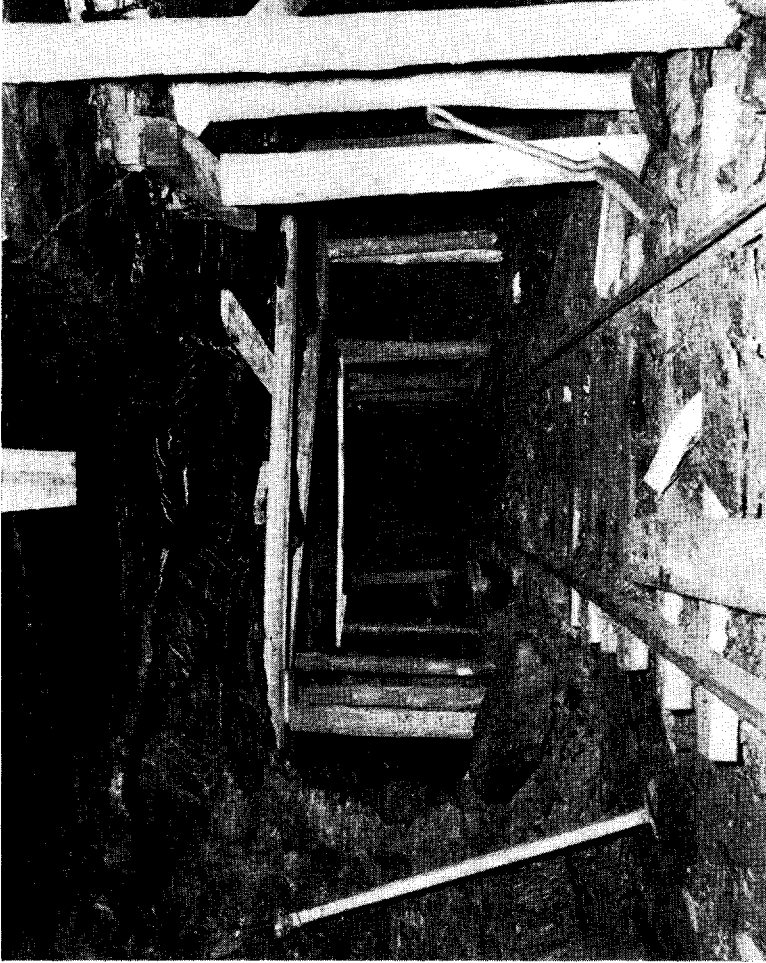
Scene of fatal accident to John Clark, George's Creek Coal Co., Inc., Lonaconing, Allegany County, September 11, 1947.
