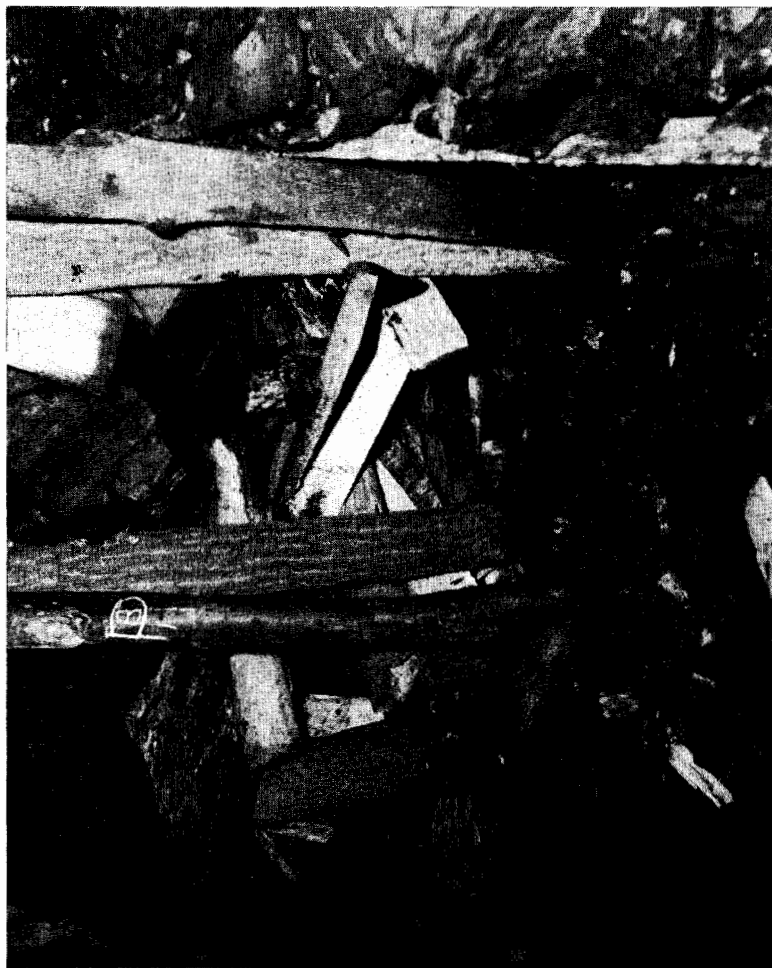
Scene of fatal accident to Charles Carlyle Conner, Conners-Haines Coal Co., Lonaconing, Allegany County, August 1, 1947.
