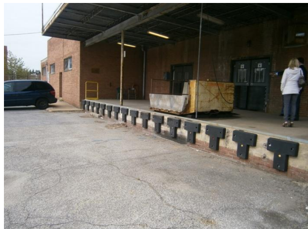
Photograph 46. Loading dock along northeastern portion of the US Post Office building.
