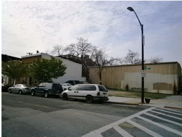
Photograph 1. Northwestern portion of the Site (127 to 145 West West Street).
