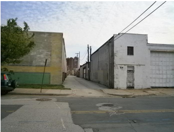
Photograph 55. ABC Box Company, Creek Alley and Baltimore Toolworks adjoining the Site to the north.
