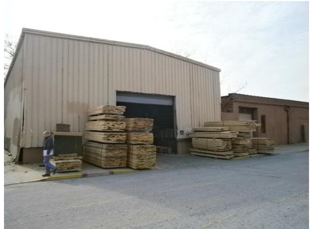
Photograph 2. Metal lumber shed in northwestern portion of Furst Brothers (1203 to 1223 Leadnehall Street).
