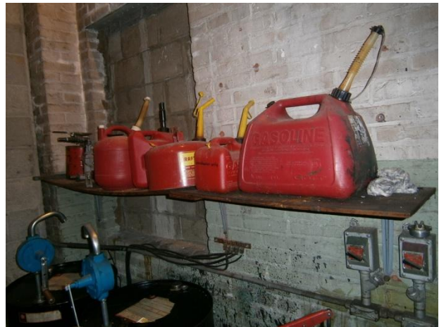
Photograph 34. Gasoline cans in northwestern portion of the air compressor room.
