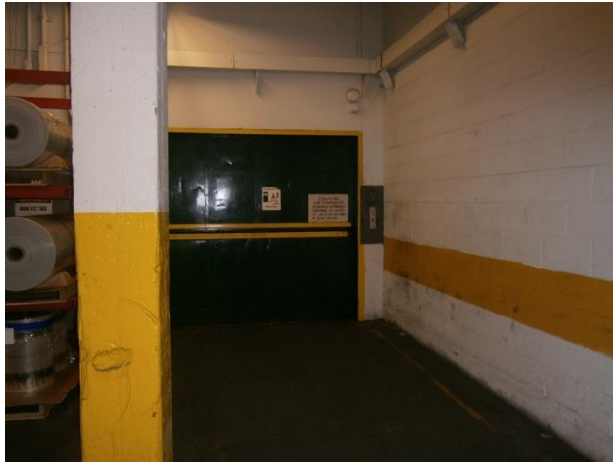
Photograph 35. Freight elevator in western portion of the southern VacPac building.
