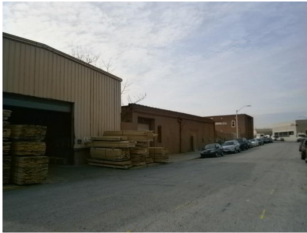
Photograph 3. Western portion of the Site (Furst Brothers).
