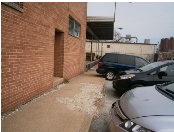
Photograph 45. Eastern portion of the US Post Office building.
