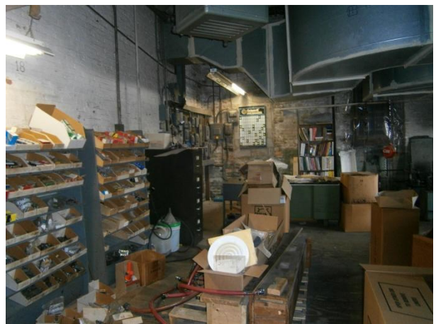
Photograph 40. Second floor storage in northern portion of the southern VacPac building.
