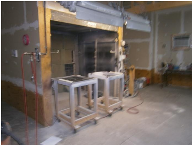
Photograph 21. Finishing paint booth in central portion of the Furst Brothers building.
