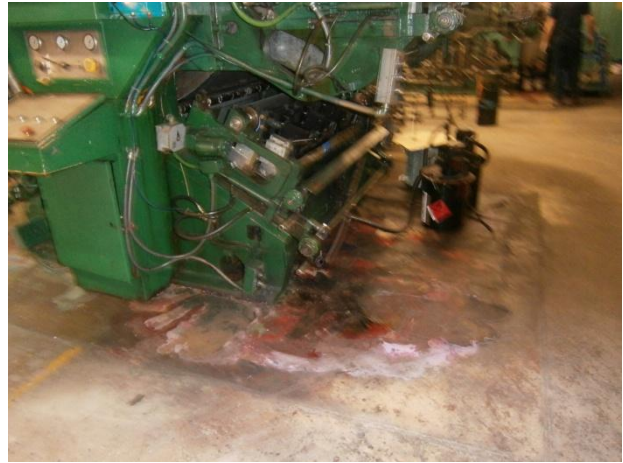
Photograph 30. Ink storage and minor concrete staining along printing machines in central portion of the northern VacPac building.
