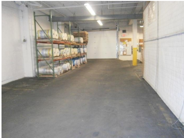
Photograph 37. First floor storage in southern portion of the southern VacPac building.
